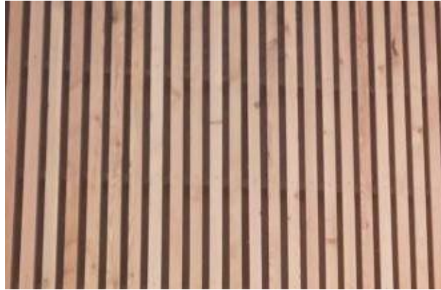
Open joint vertical timber cladding (east elevation)
