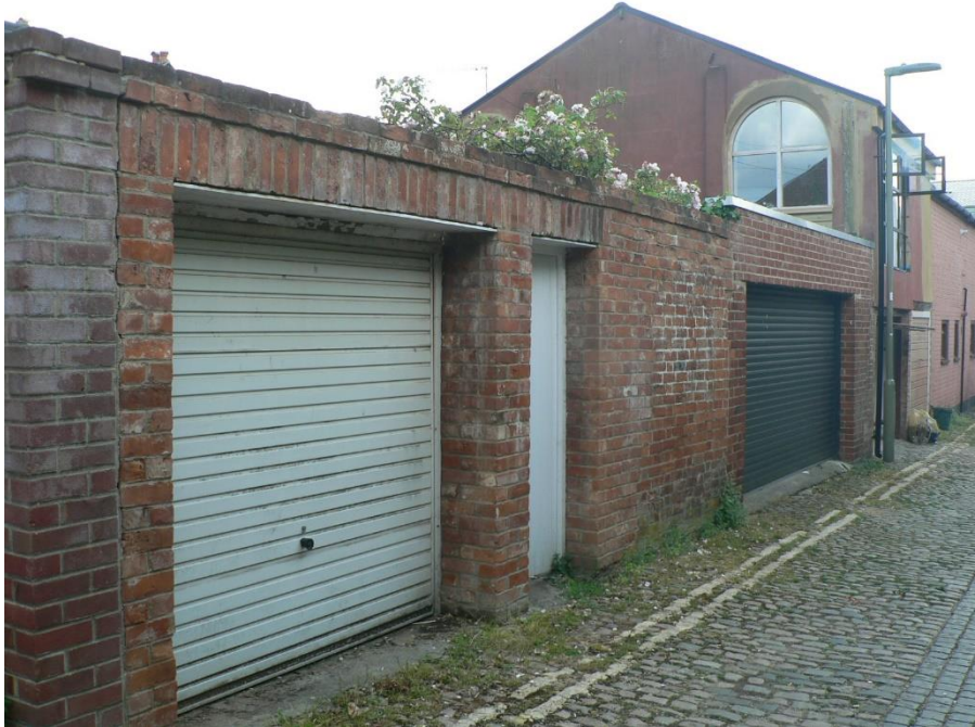
Existing rear elevation (Walton Lane) showing garage and pedestrian doors
