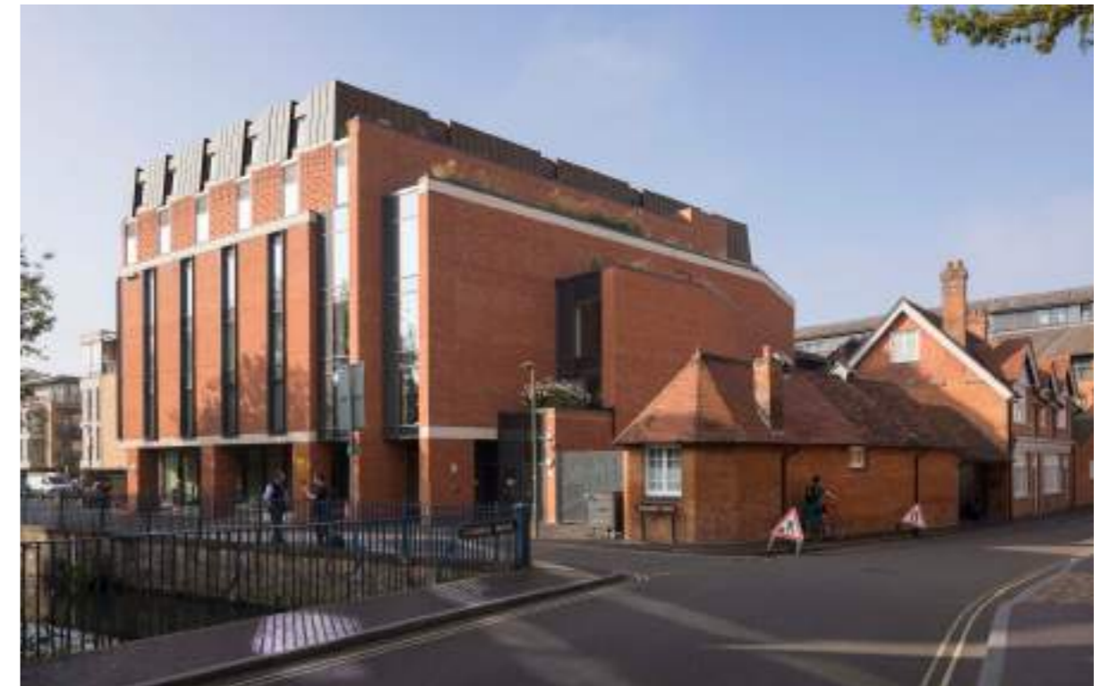
VIEW FROM QUAKING BRIDGE - OTHER AMENDMENTS (FINAL VIEW)
