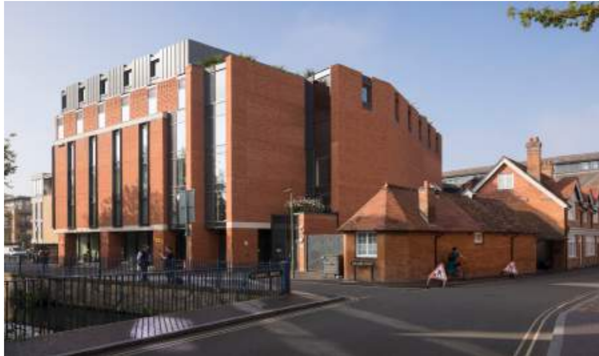
VIEW FROM QUAKING BRIDGE- PRE-PLANNING APPLICATION
