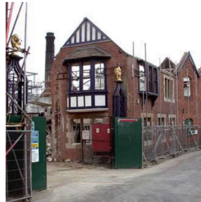
Figure 3.7 Works to convert the lion gate brewery after its closure in 1998
