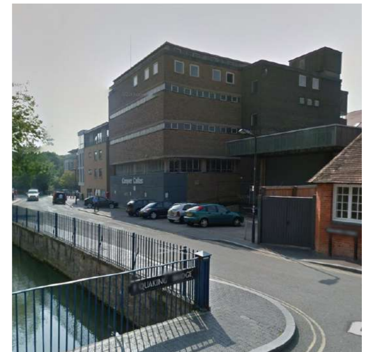
Figure 3.8 The Cooper Callas Building before deomlition (2016)
