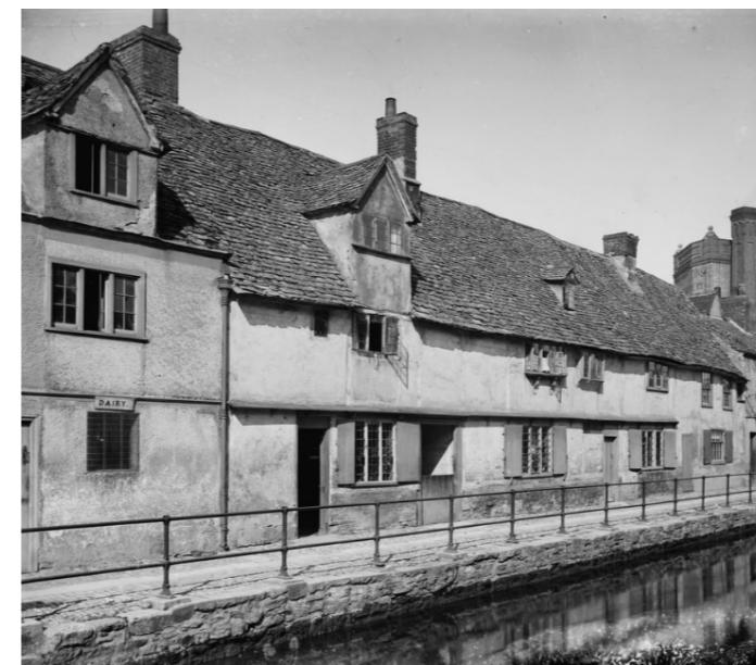
Figure 3.3 The 16th-17th Century cottages on Fisher's Row with Brewery buildings visible behind
