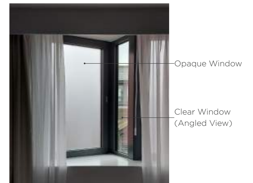
EXISTING INTERNAL VIEW (4TH FLOOR)
