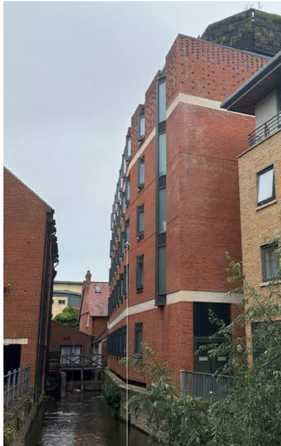
The existing window treatment on Wareham façade prevents any overlooking into the opposite residential properties. A combination of angled windows and opaque glazing provides sufficient light into the rooms, whilst reducing inter-visibility between the two buildings.
