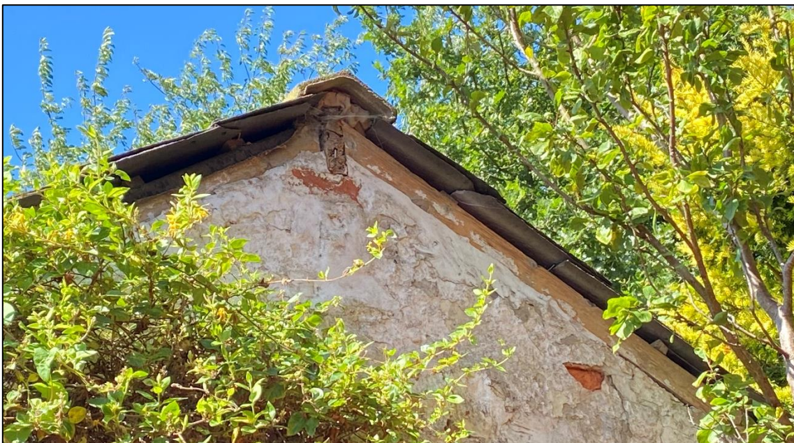
Plate 8: Verges of the outbuilding had large gaps apparent offering potential roost features and offering access into the internal spaces.
