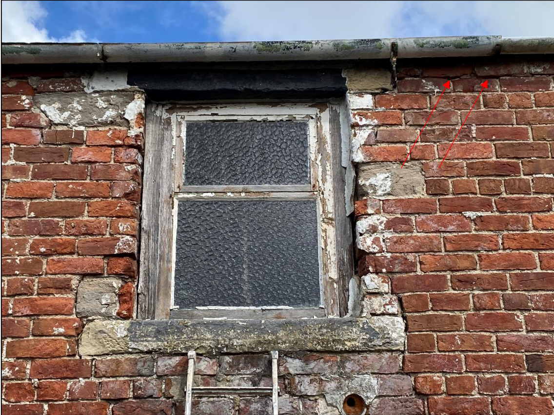
Plate 26: During construction, gaps will be incorporated into the brickwork that are suitable for crevice dwelling species and are similar to the existing gaps.
