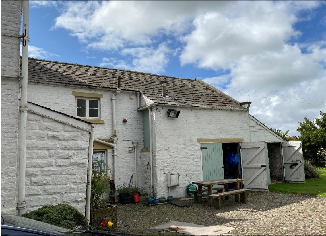
Plate 1: General view of the rear of the building.
