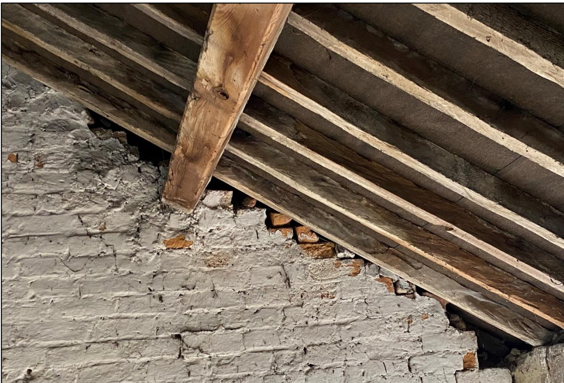
Plate 20: Gaps were apparent on top of the gable wall of the barn, offering PRFs.
