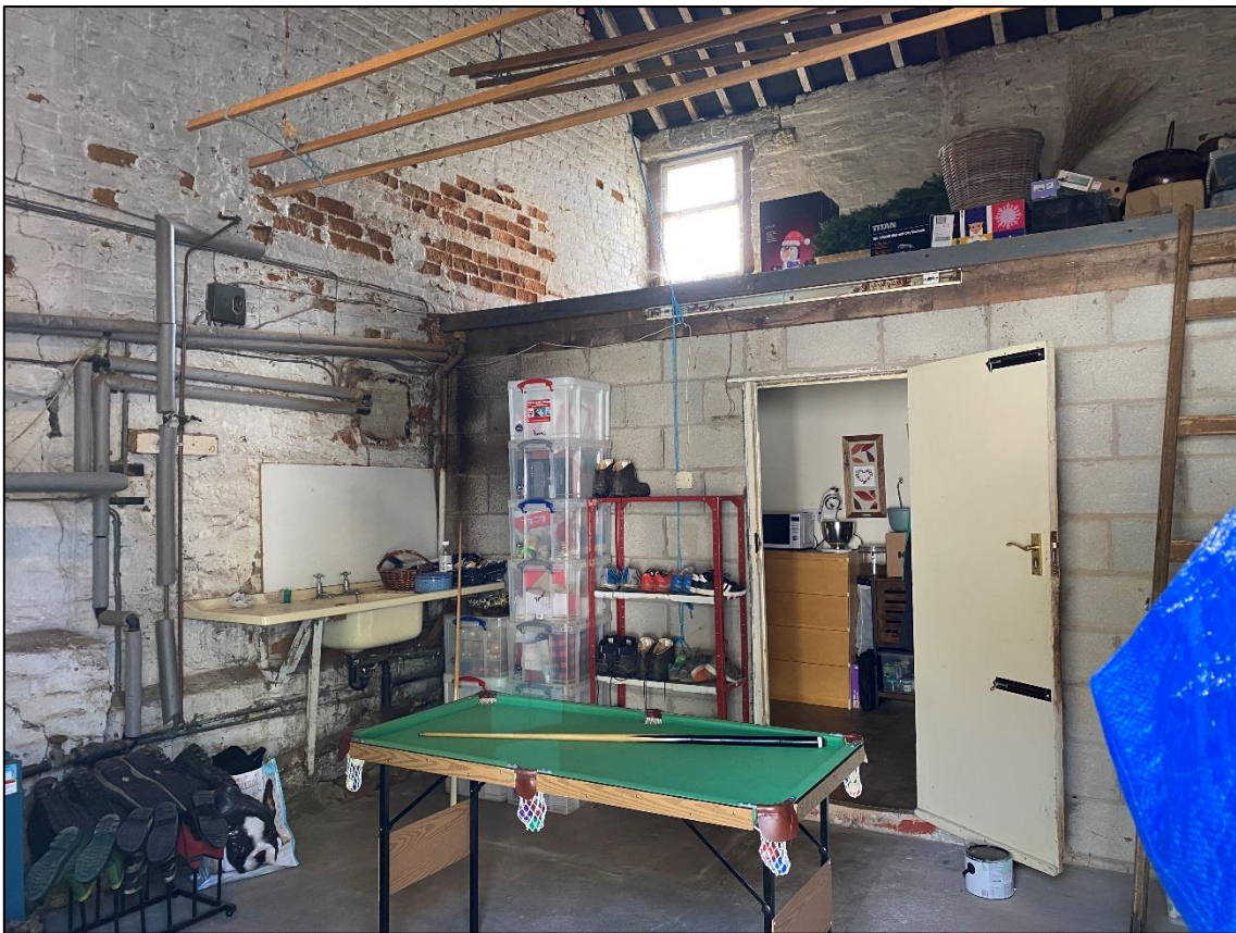
Plate 14: The rear barn consisted of a single open internal space which was in-use and accessed via the kitchen.
