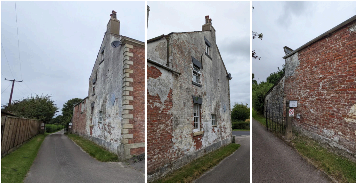
Exposed and weathered south (side) elevation of the Olde Ship, photographed Aug.2022
