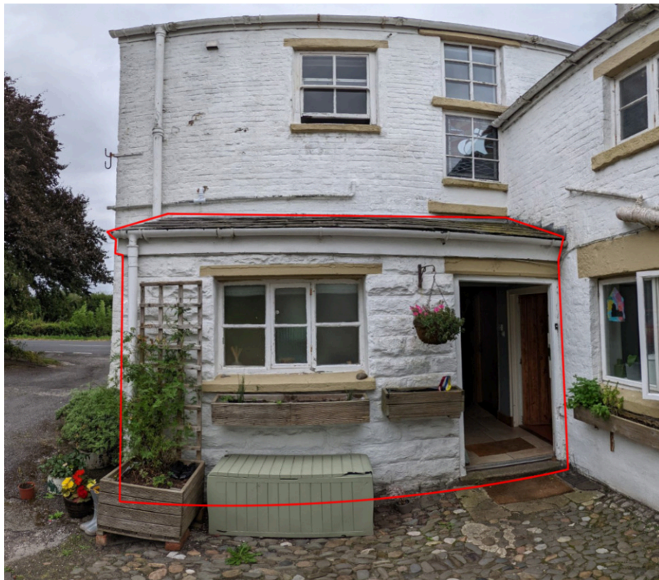
Proposed single Storey Lean-to, proposed to be demolished, photographed Aug.2022
