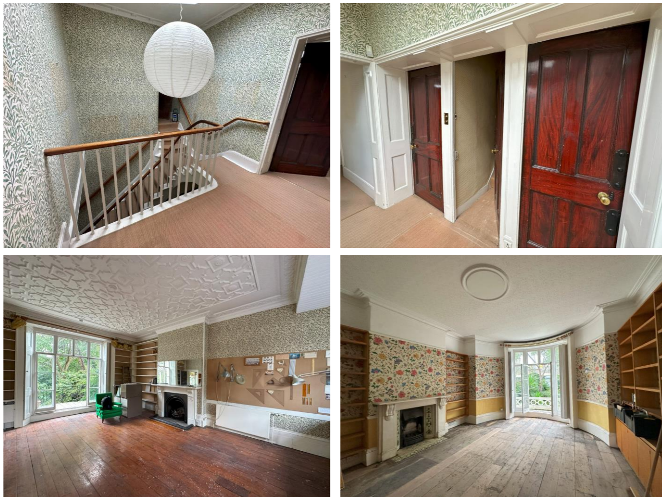
Figures 29-32 clockwise from top left): The 1 st floor landing, door to the secondary staircase, the ground floor room within the former stable block and the main rear room at ground floor level.
