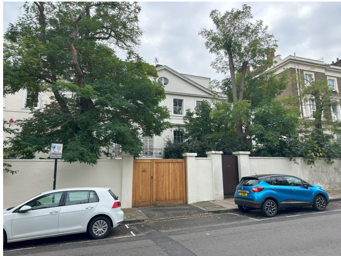
Figure 1: The front façade of the house, setback from Greville Place behind a tall front boundary wall.
