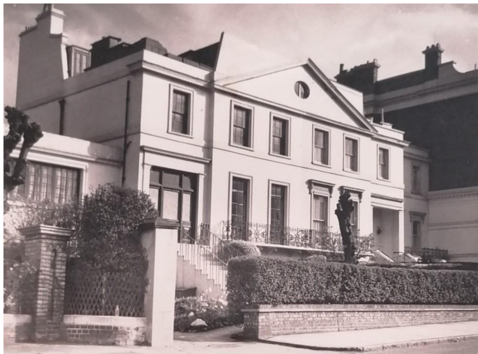
Figure 9: The semi-detached pair of houses at nos. 20 (left) and 18 (right) in 1959 [© City of Westminster Archives Centre T138 (2a)]. Note the surviving stable block to the side of no.20, albeit converted, whereas this element had been extended upwards at 1 st floor level on no.18 by as early as 1915.
