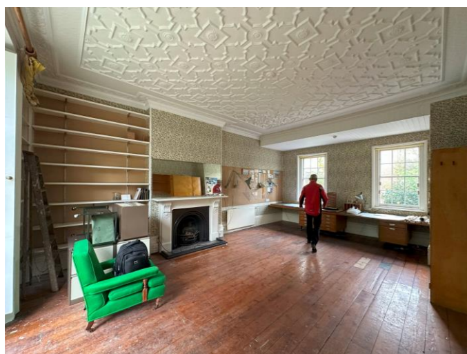
Figures 39-41 (clockwise from top left) The front wall at ground and 1 st floor levels, and within the 1 st floor of the former stable block.
