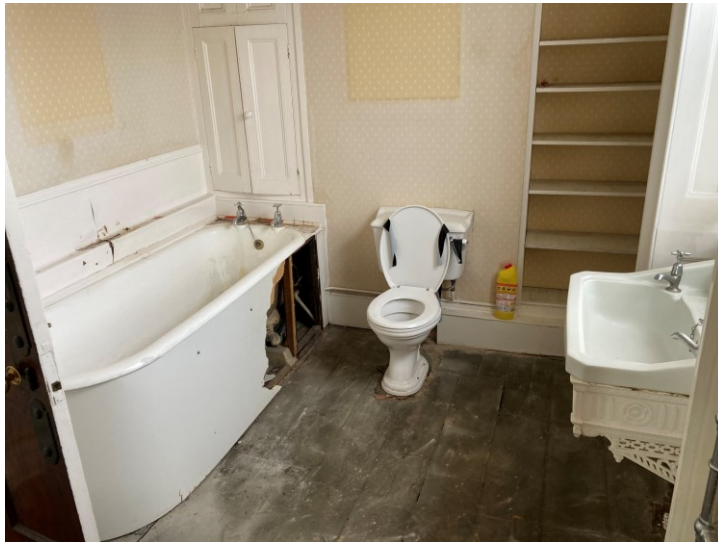
The first floor family bathroom (2) condition as existing
