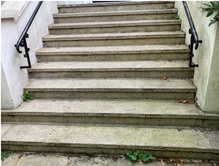
ENTRANCE STEPS TO FRONT DOOR MAIN ENTRANCE.
