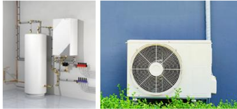
Figure 7: Left to right typical air source plant room installation, typical outdoor small fan unit, example cover for aesthetic purpose
