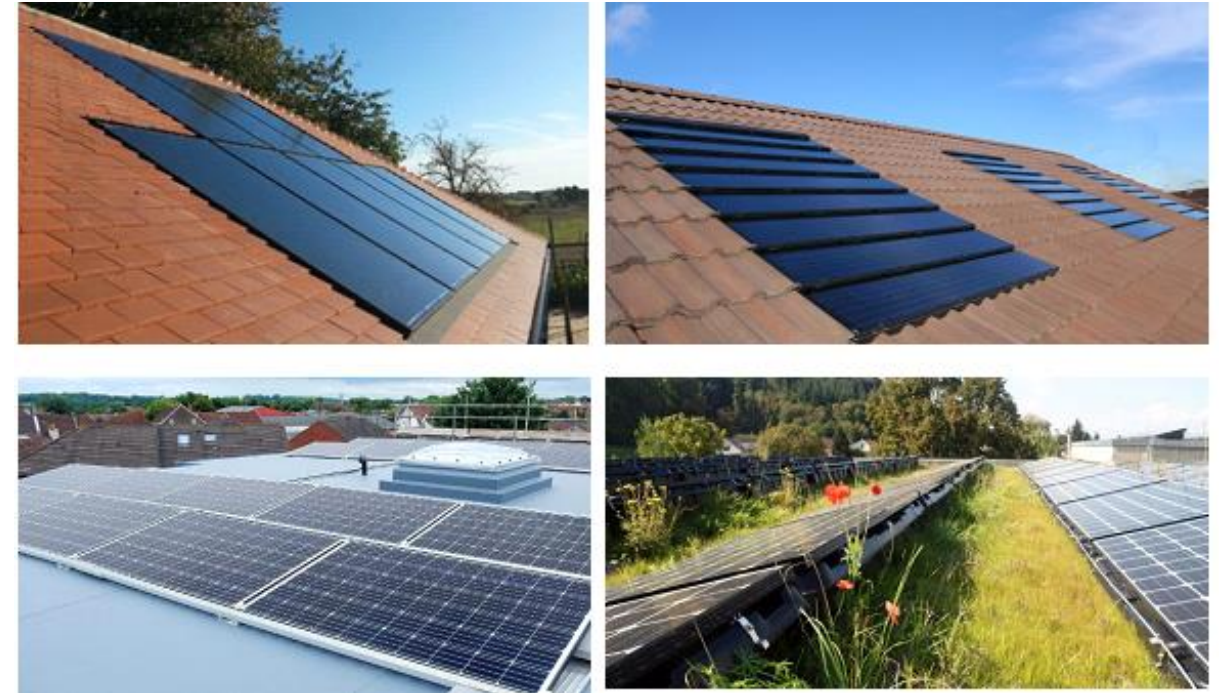
Figure 9: Solar installation examples clockwise from top left: In roof, tile in-roof, typical flat roof, flat green roof
