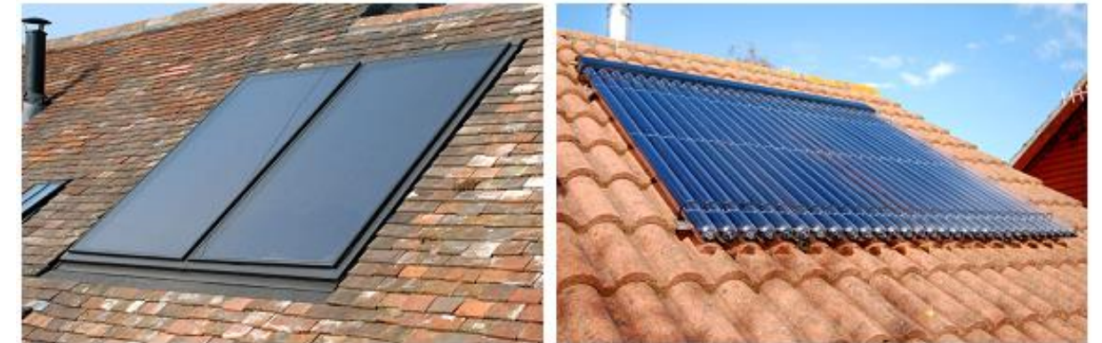
Figure 16: Solar thermal installation examples left in-roof, right - vacuum tube
