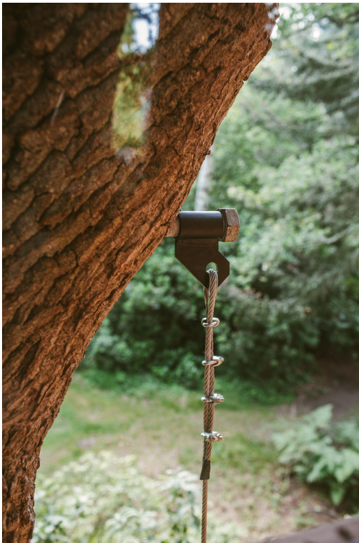
Cable suspension in conjunction with a TAB on the main beam, provides additional strength to the TAB.
