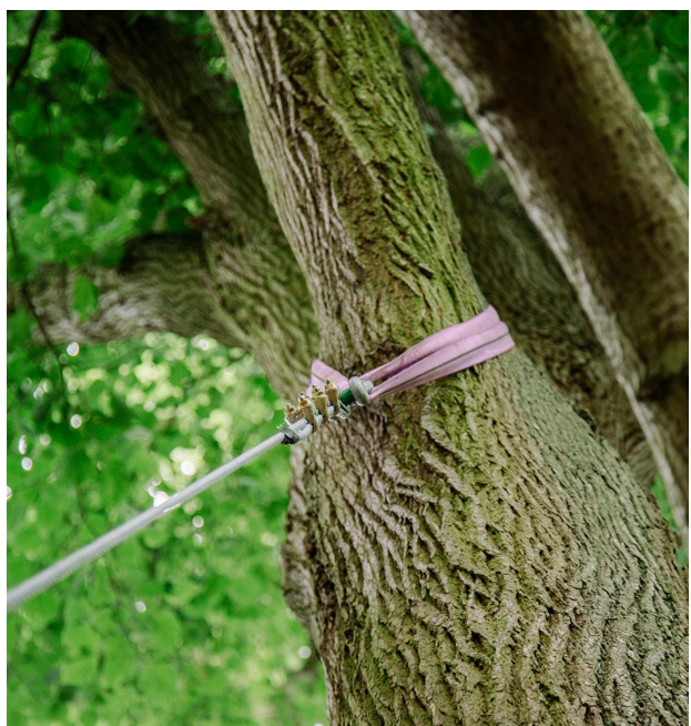
Images showing how a suspension attachment is made with a cargo belt.
