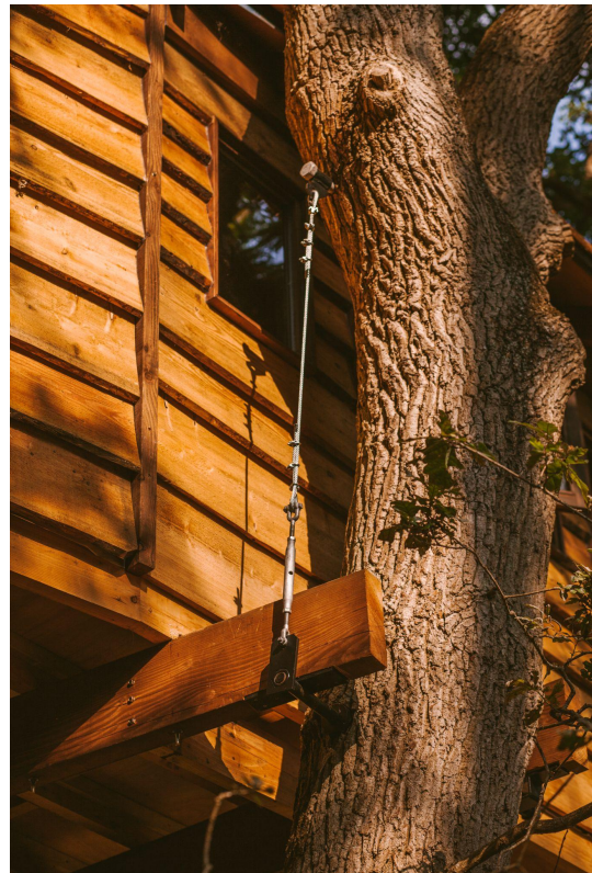
Cable suspension in conjunction with a TAB on the main beam, provides additional strength to the TAB.
