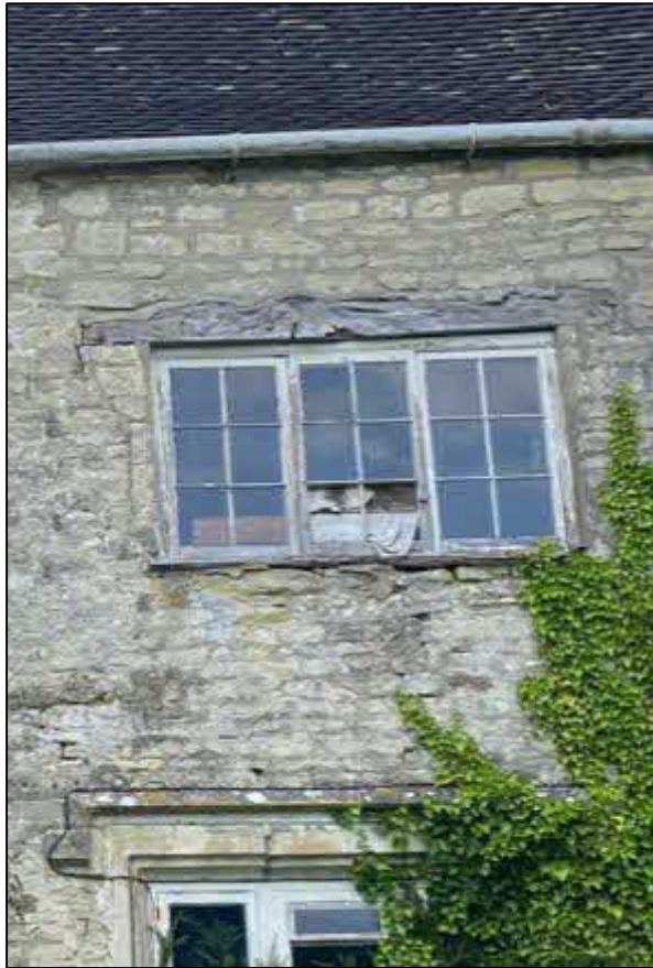
Figure 31 Timber window lintel
