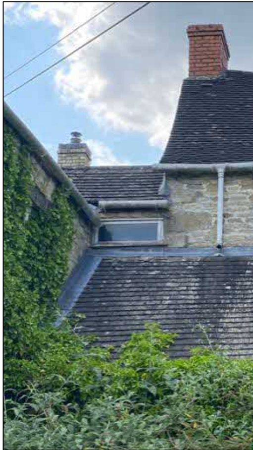
Figure 29 Photo showing lead flashing
