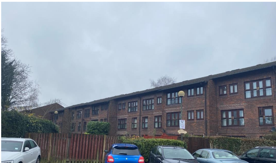
Plate 4.2: Overview of B1 Building (Eastern Elevation)
