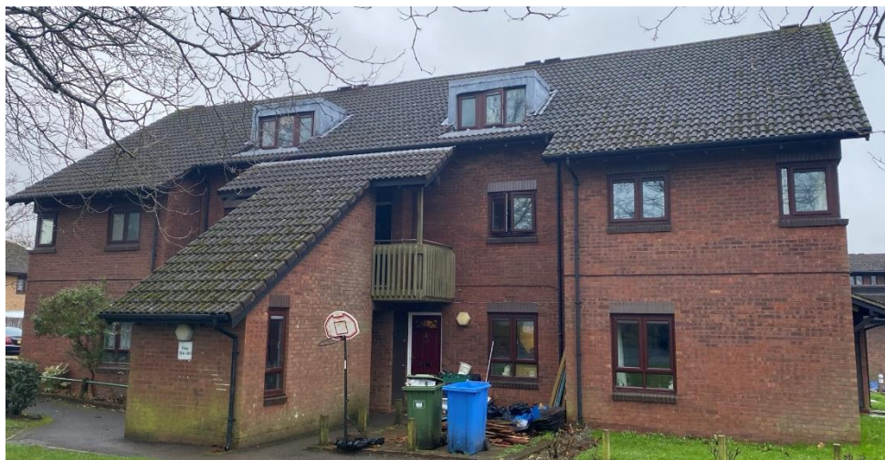
Plate 4.10: Overview of the Northern Elevation
