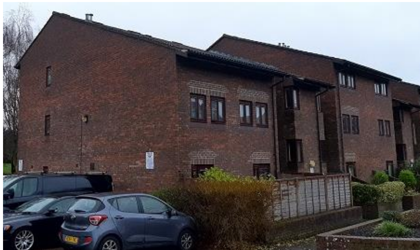
Plate 4.5: Overview of B2 Building (South-Eastern Elevation and Part of Northern Elevation)
