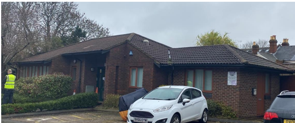
Plate 4.14: Overview of B5 Building (Southern Elevation)
