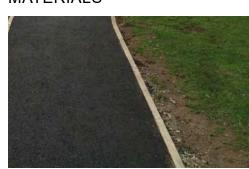
(A) MACADAM FOOTPATH. SUPPLIER: TARMAC OR EQUAL. SUB-BASES TO BE **TESTED ON SITE PRIOR** TO INSTALLATION TO DETERMINE SUITABILITY. INSTALLED TO SUPPLIERS RECOMMENDATION.
