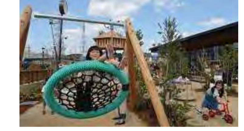
7 BASKET SWING. SUPPLIER: TIMBERPLAY. PRODUCT: 'CRADLE NEST' (6.14520) OR EQUAL APPROVED. TIMBER AND GALVANISED STEEL CONSTRUCTION. INSTALLED TO SUPPLIERS RECOMMENDATION.
