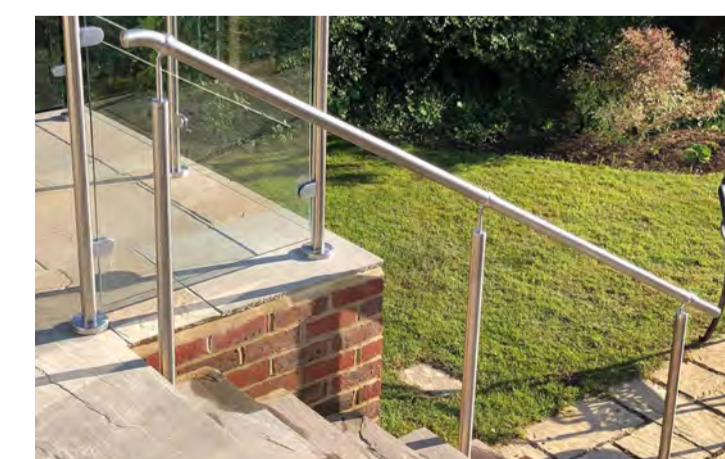
F HANDRAIL. TO BE GRADE 316 STAINLESS STEEL WITH SATIN BRUSHED FINISH. HEIGHT ABOVE PITCH LINE TO BE 900MM. HANDRAIL TO BE 50MM DIAMETER WITH ADDITIONAL LOWER HANDRAIL FOR EXTRA SUPPORT IF REQUIRED. TO BE MOUNTED TO STEP SURFACE USING STAINLESS FIXINGS WITH COVER TO FABRICATORS SPECIFICATION.
