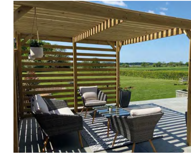
G PERGOLA. 7.8M X 3.6M CONSTRUCTED USING HARDWOOD TIMBER. POSTS: L:2750MM X 150MM X 150MM ROOF STRUCTURE: L:VARIOUS X 150MM X 50MM ROOF SLATS: L:2400MM X 50MM X 50MM COLOUR COORDINATED VERTICAL TIMBERS: L:2650MM X 50MM X 50MM PAINTED TO MATCH COLOURS OF ENTRANCES.
