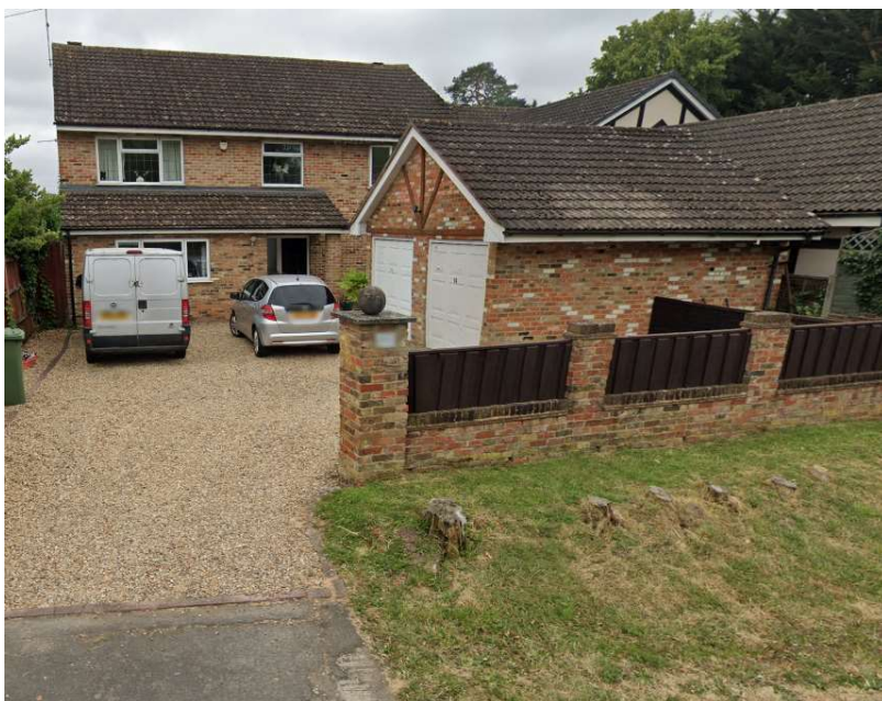
Garage to front of house in North Street
