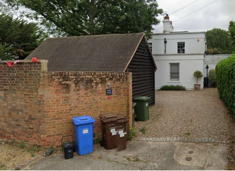
Garage to front of house in North Street
