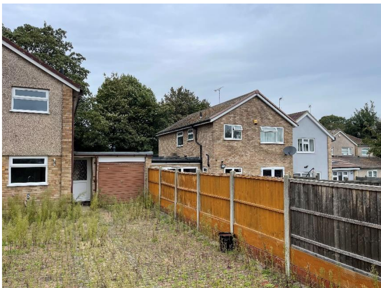
Fig 7 Rear View of 51 Finch Lane showing neighbour no.53
