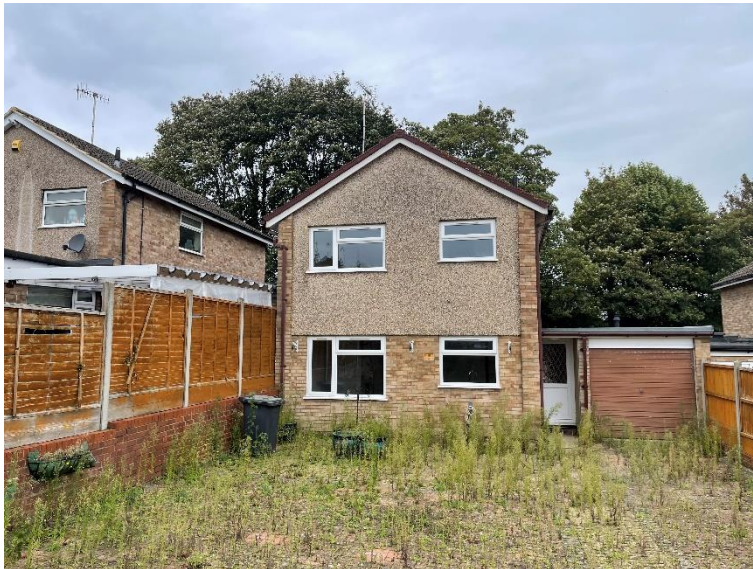
Fig 6 Rear View of 51 Finch Lane showing neighbour no.49
