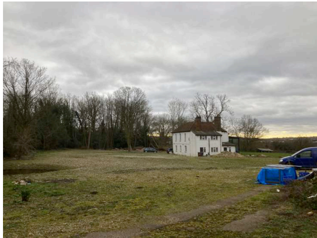
PS-01 E-View looking in a south easterly direction across the site.
