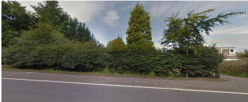
Site of “Seacroft” streetscape prior to demolition – active travel route shown.
