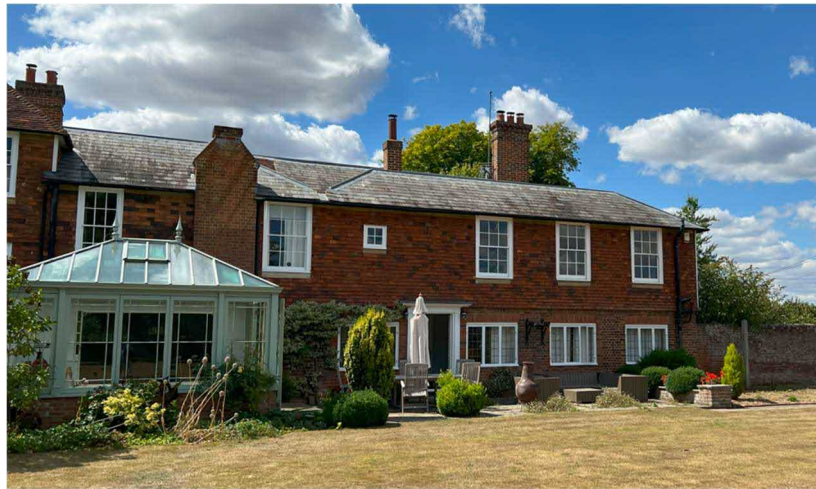
Fig 1: Rear Elevation of Laddingford House showing the Conservatory to be removed
