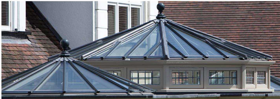
Fig 11: Aluminium, glass, lead roof lanterns by Vale Garden Houses
