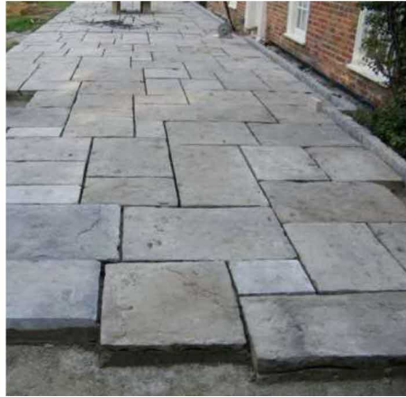
Fig 15: Reclaimed York being laid
