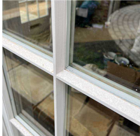
Fig 8: External window detail
