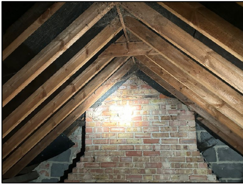
Figure 9 – General view of the roof void looking west towards the chimney
