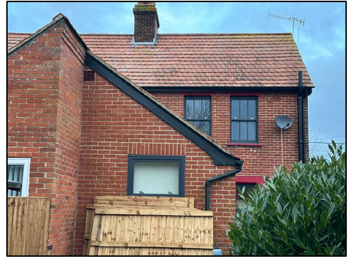
Figure 4 – Rear of the property showing the single-storey extension
