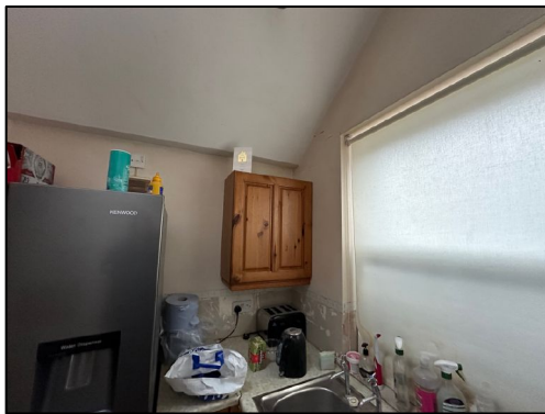
Figure 11 – Internal section of the extension to be removed
