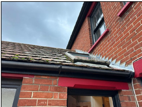
Figure 5 – Junction of the extension of which attaches to the main house
