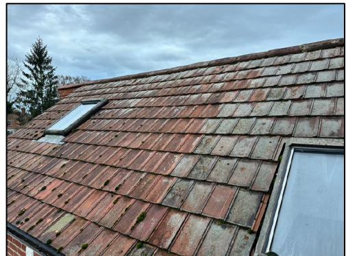
Figure 6 – Roof to the extension
