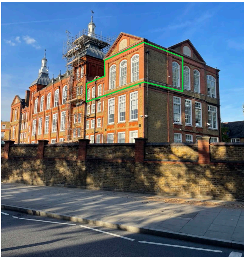
West (facing Kennington Road) and South Elevations (facing Stannary Street ) - flat 26 marked by green outline.
