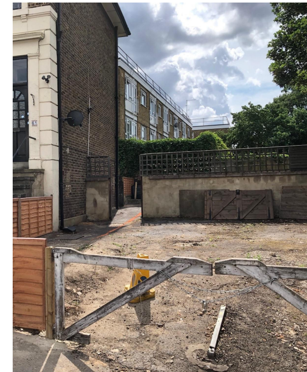
Existing Site View
