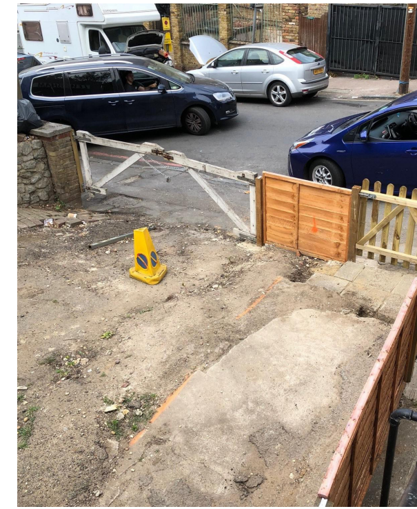
Existing Site View
