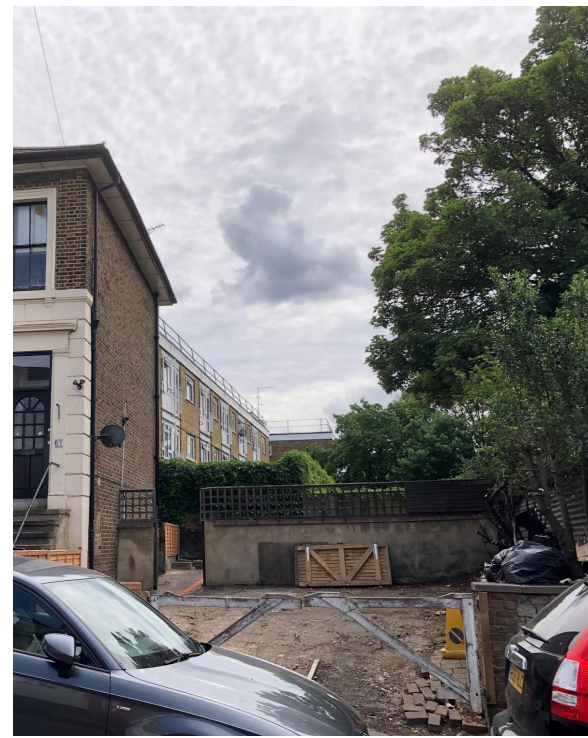
61 Marischal Rd Flank Wall and Site View
