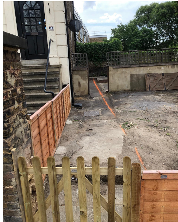
Existing Site View
