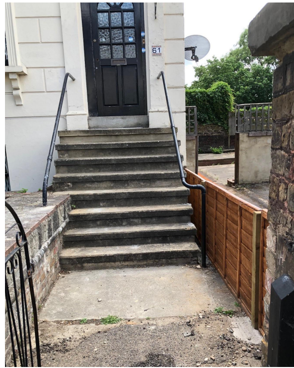
61 Marischal Road Main Entrance View
