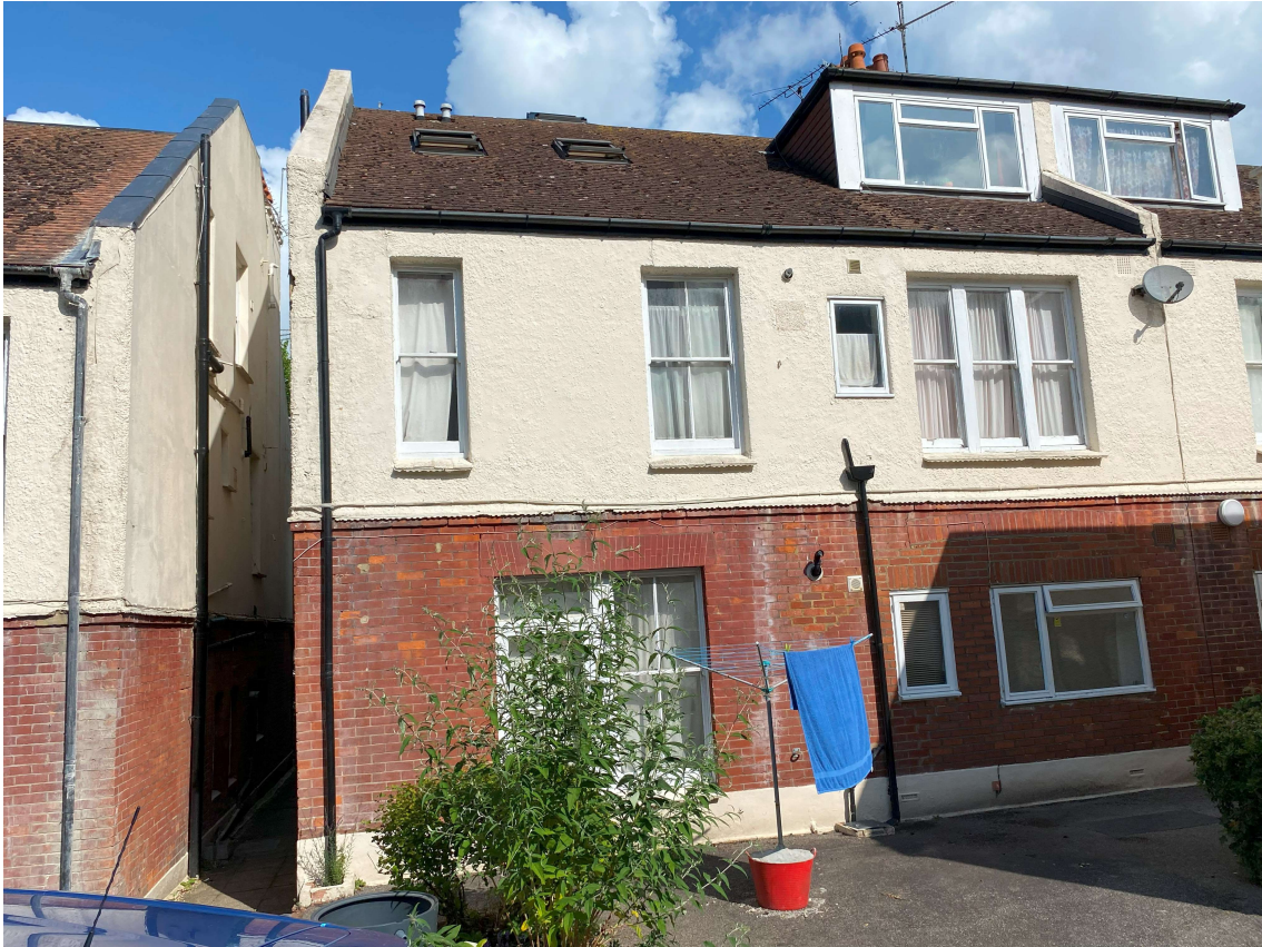
Rear elevation No 26 Windlesham Gardens
