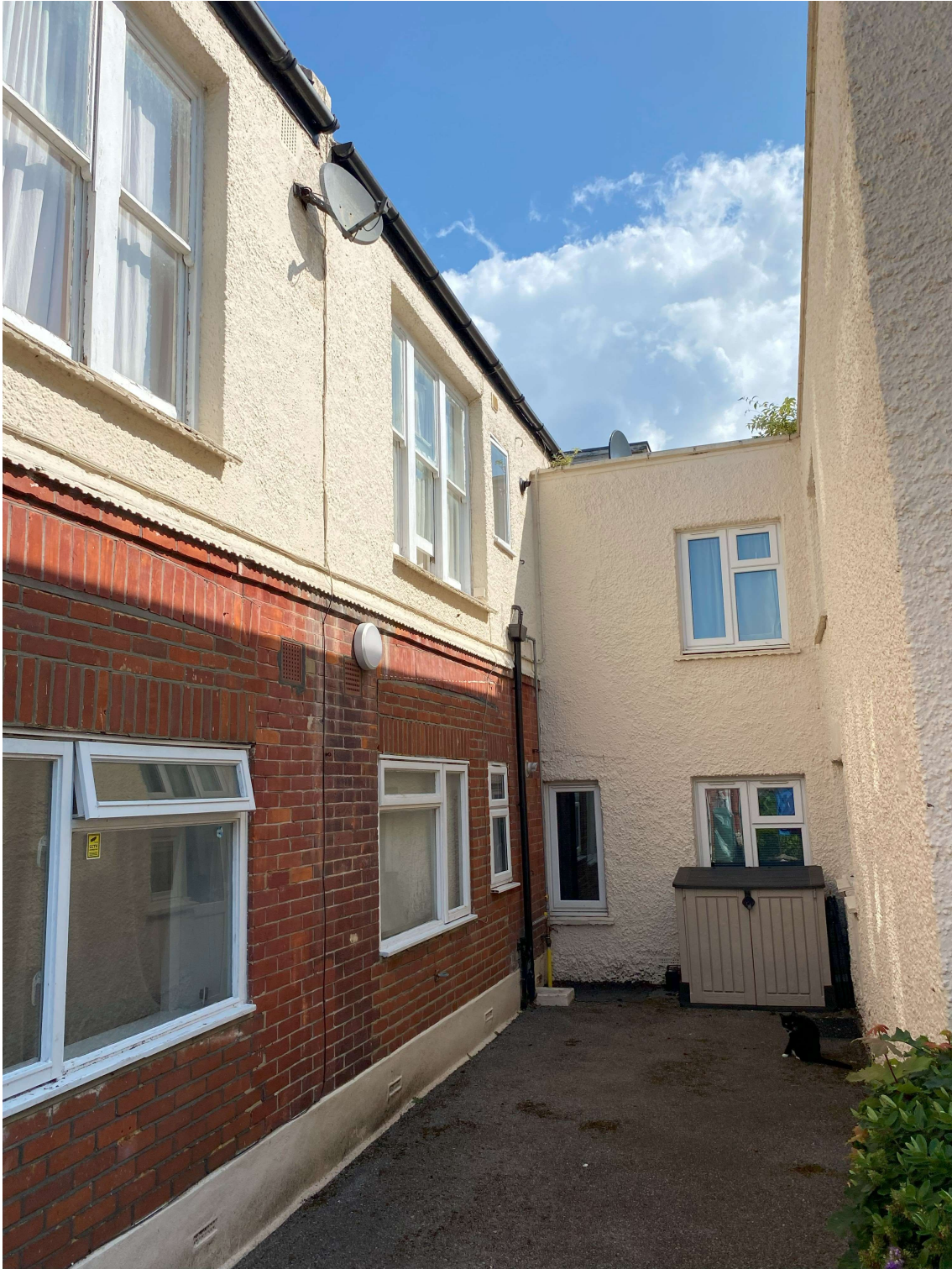
Rear elevation No 28 Windlesham Gardens
