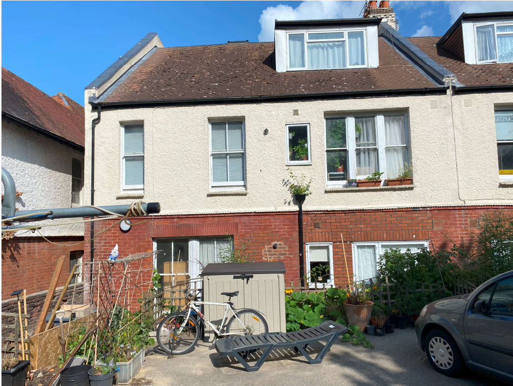
Rear elevations No 22 Windlesham Gardens
