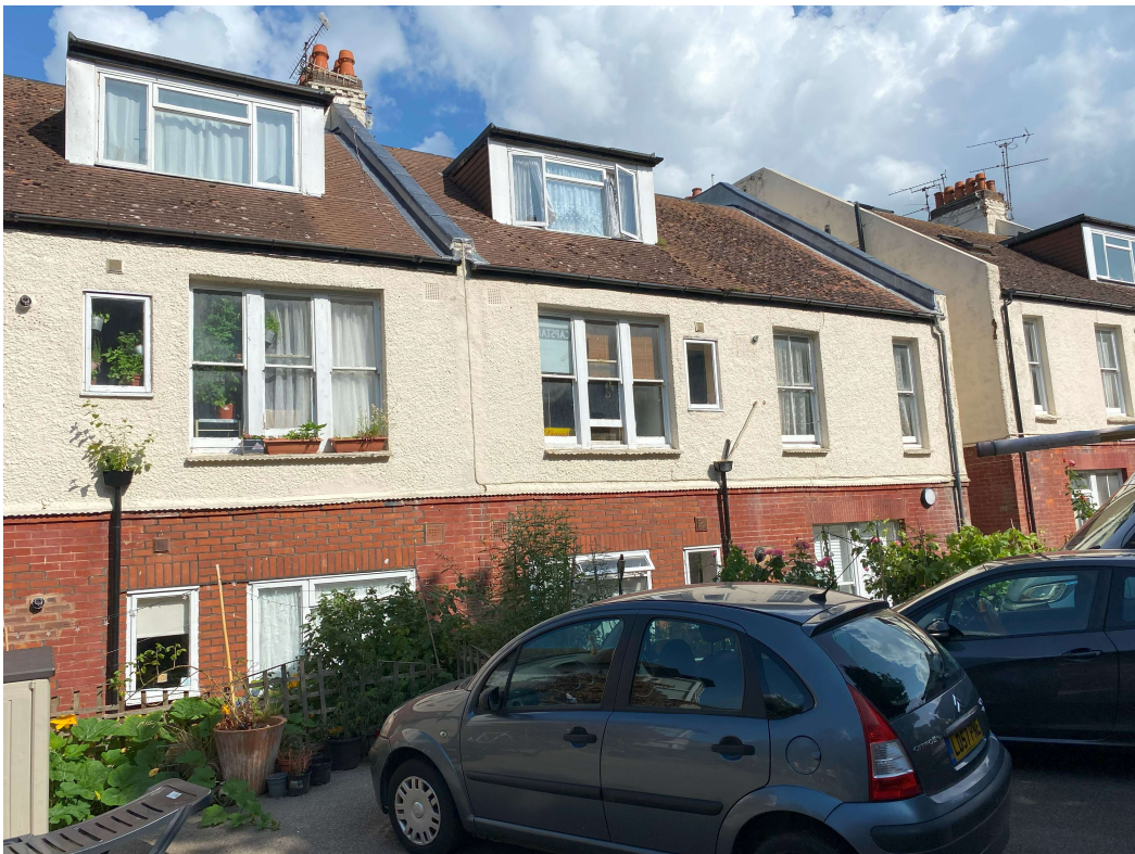
Rear elevation No 24 Windlesham Gardens
