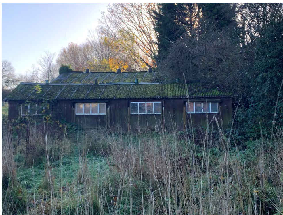
Photo 4) Looking South from rear of bungalow on site towards wooden shed (brick shed behind) with asbestos roof.
