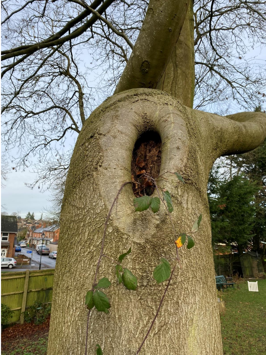
SAL6 T7 beech with cavity on the tension / upper side of the bend.
