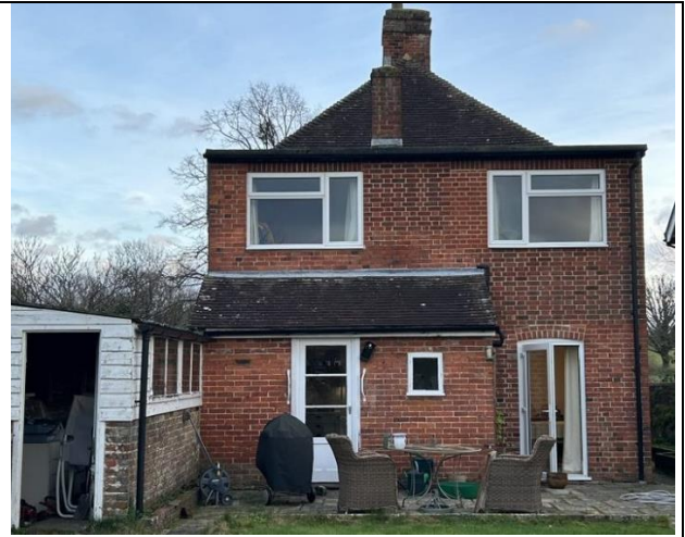
Photograph 2: North West elevation of house
