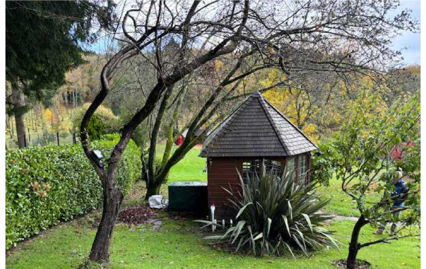
Existing swimming pool pump building
