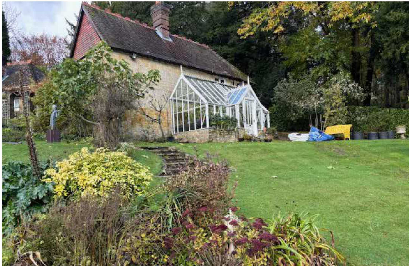
Existing greenhouse and two storey building.
