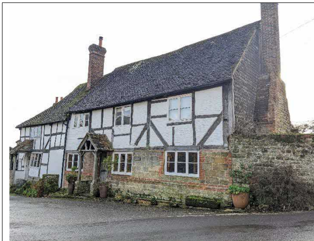
Photograph 1: Northern and western elevations of the house
