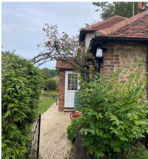
View across rear of property
