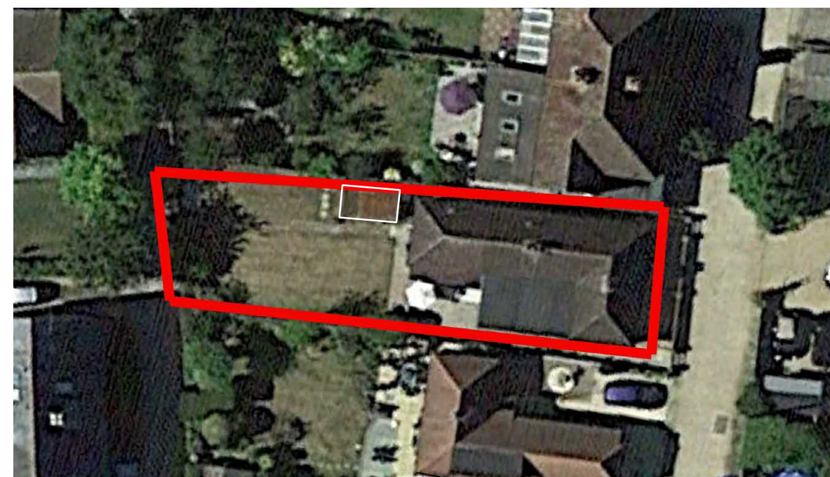
Current condition, Workshop outlined in white
