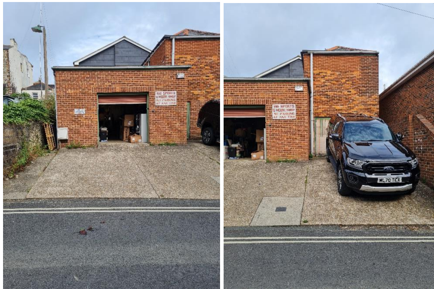
Rear of 9 Union Street facing Union Road
