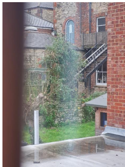
Rear of adjacent buildings
