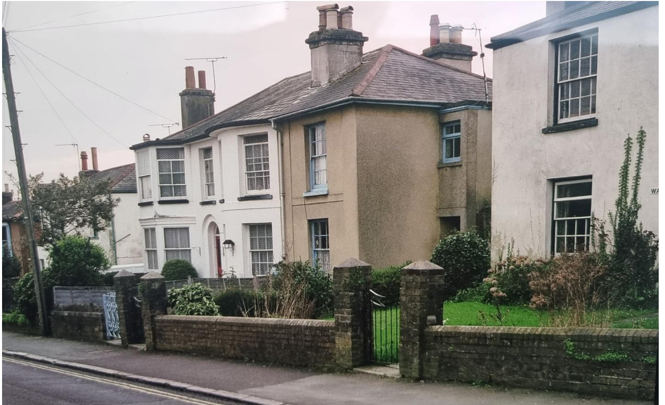
Photograph 1: 37 Melville Road in the 1960's-70's. The exterior finish is relatively new although has signs of weathering. Note the different roof tiles and the consistent render finish of the stacks
