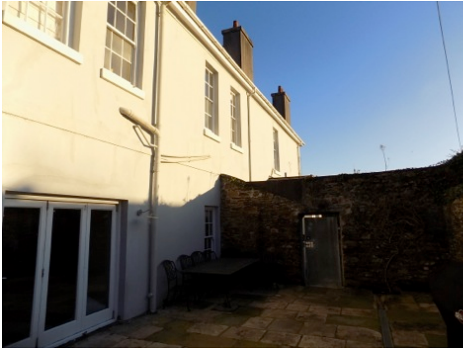
Photo 7. Bi-fold doors to courtyard from kitchen.
