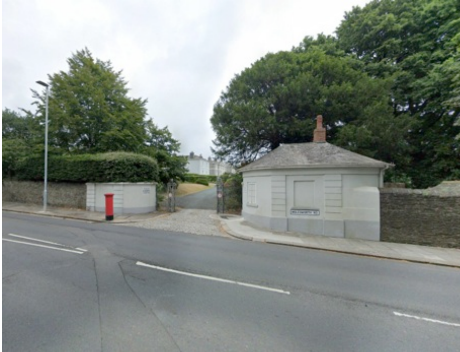
Photo 11. Lodge House and gates to Penlee Gardens.
