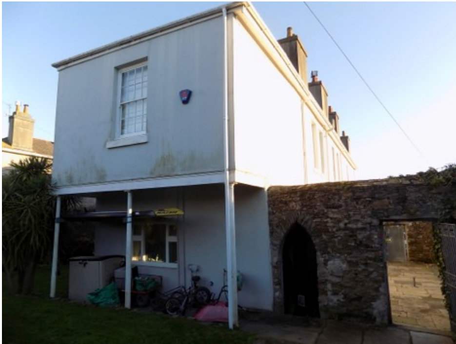
Photo 9. Rear elevation with 20th century horizontal window opening under projection of first floor bedroom.
