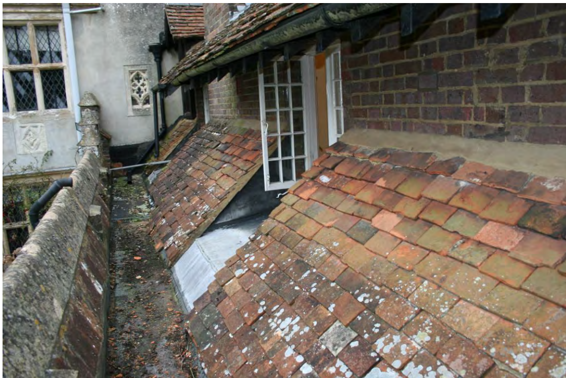
Looking N along the top of the south elevation.
