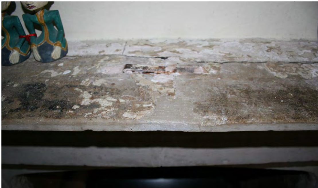
Wrought iron staple securing two halves of the fire surround.
