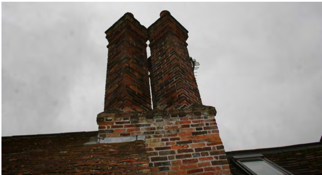
The fire stack divides into four separate shafts.
