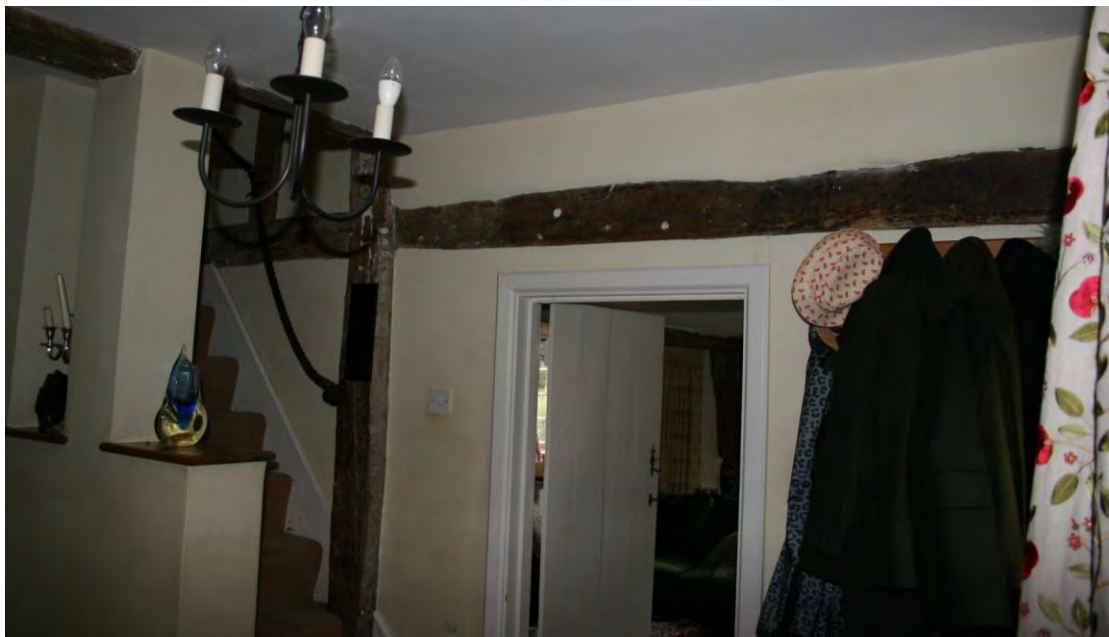
Looking E in the Lobby. The main joist is morticed for a stud wall.
