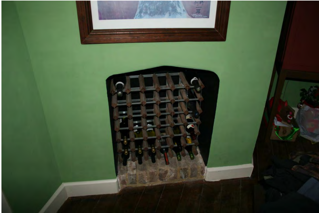
The fireplace has been given a four-centred arch.
