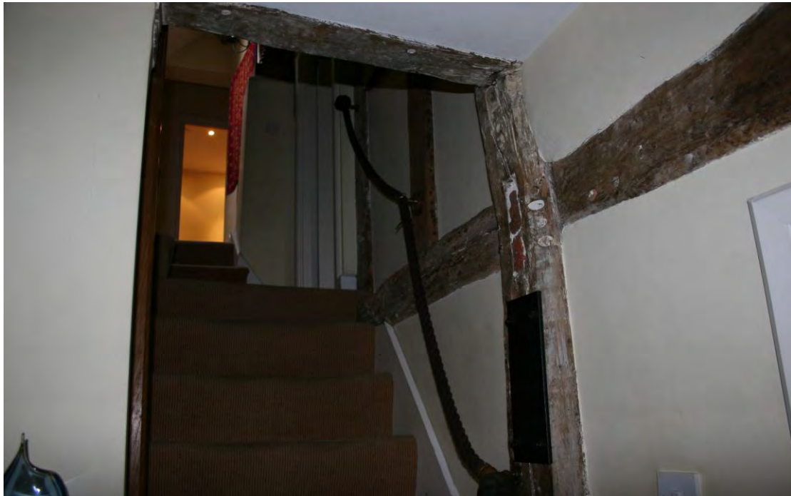
The foot of the stairs. Note the brick filled mortice and steel plate.
