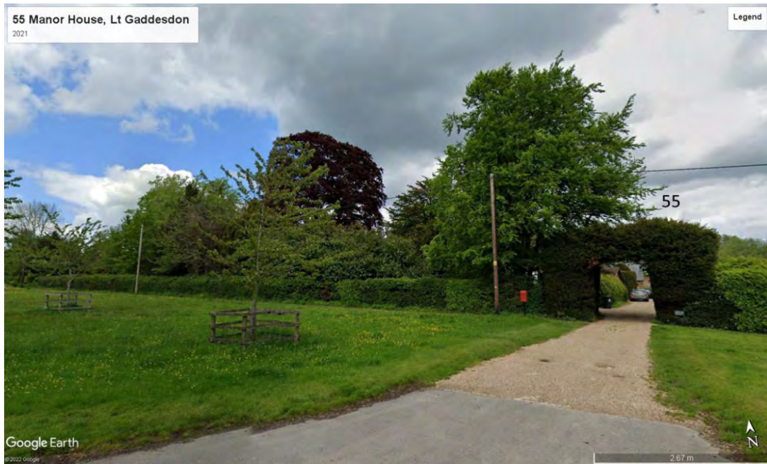
Looking NE along the drive to No55. Only the detached garage is visible.
