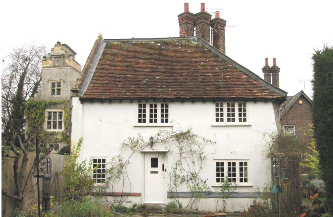
The south elevation exhibits a hipped roof with a western gable.
