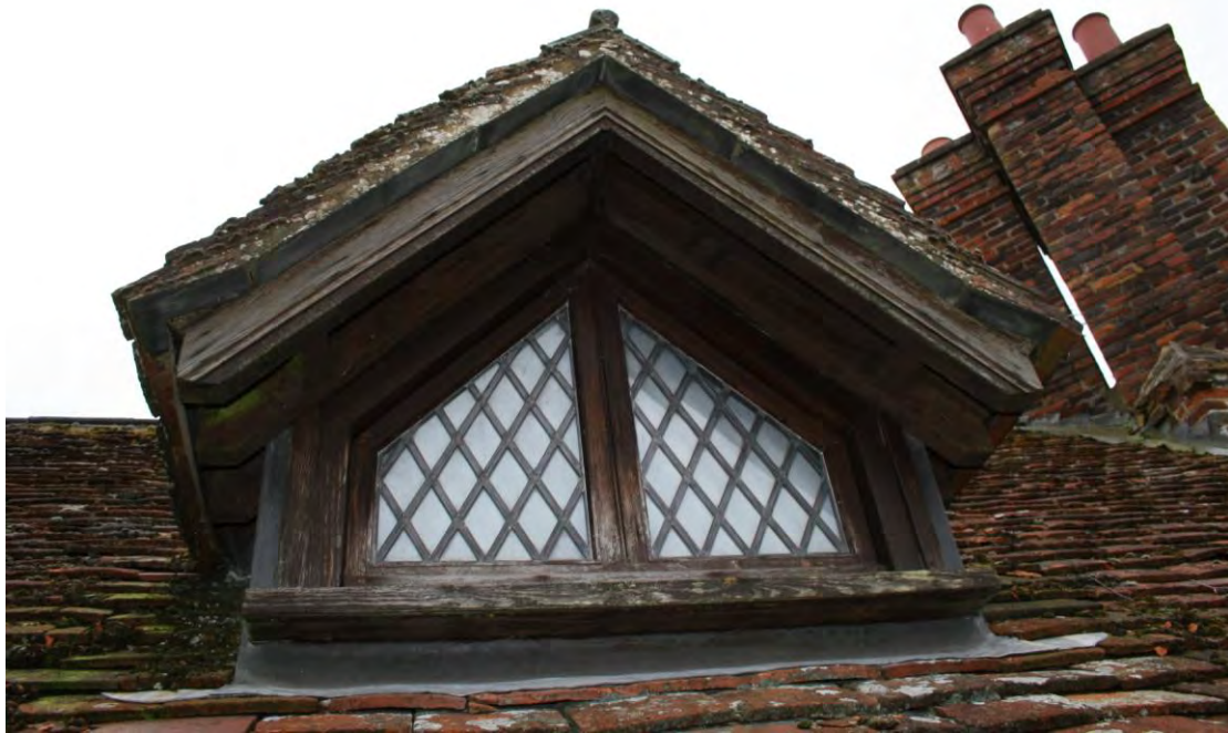
The dormer to the roof space.
