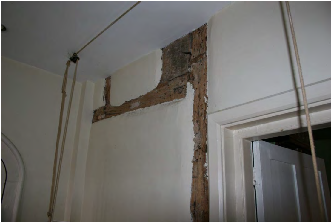
The exposed frame of the early timber range.
