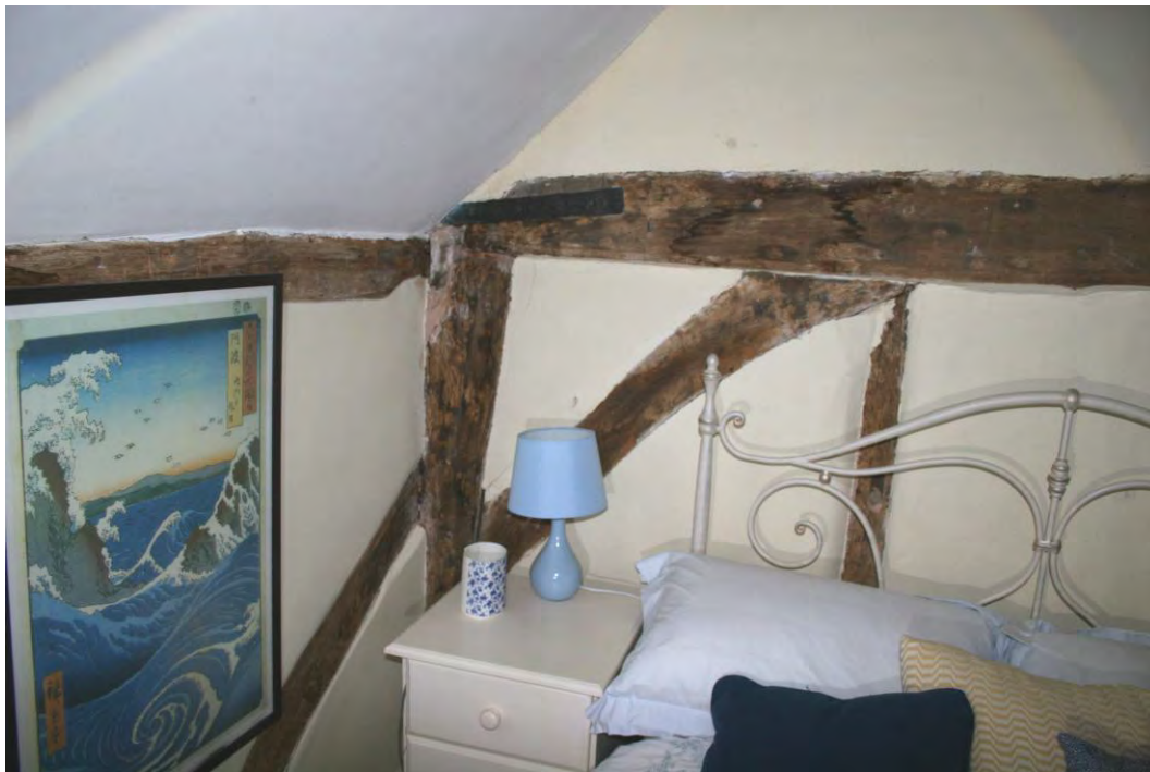
The storey post, tie-beam, spandrel and top-plate in the south and west walls.
