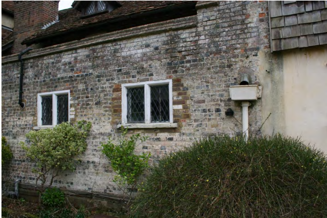
The applied facade to the south elevation. Windows appear inserted.
