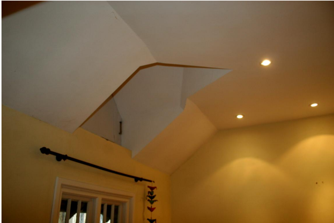
The ceiling of Bedroom 3.
