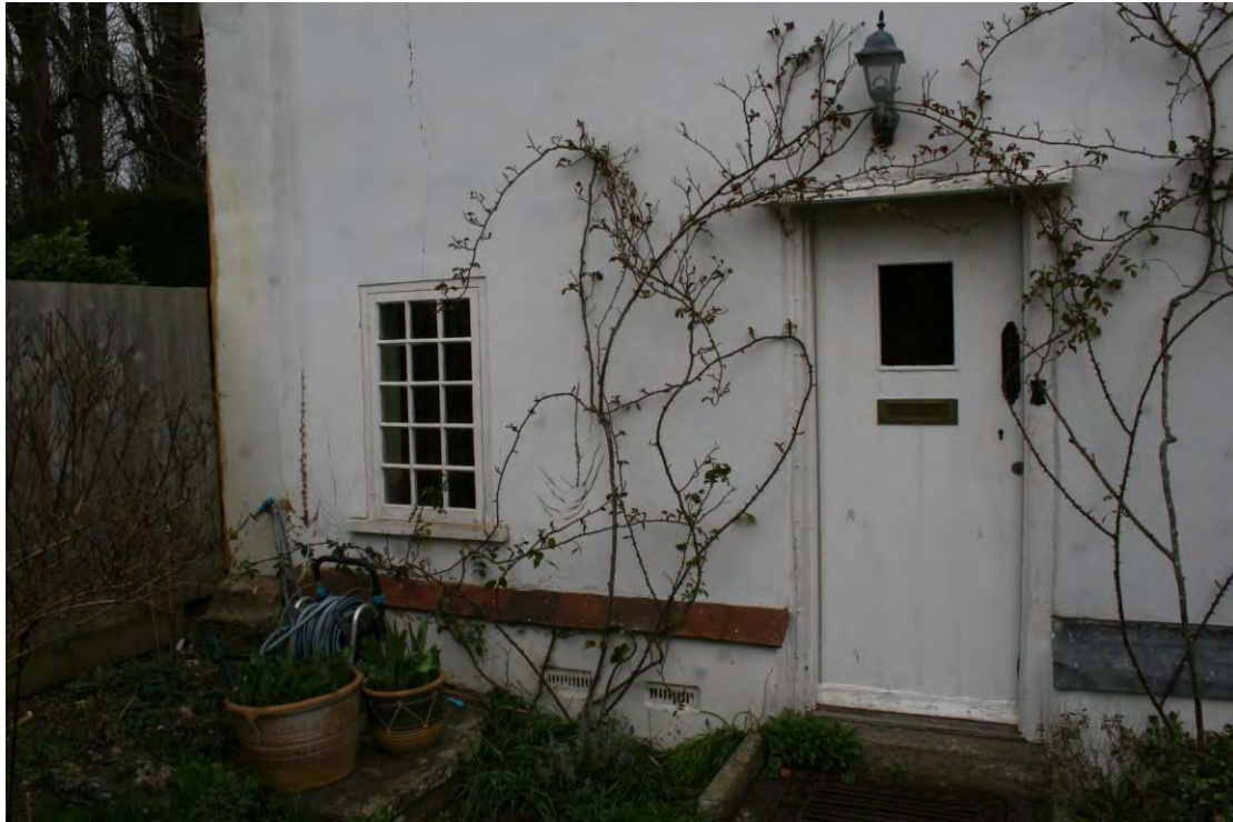
Detail of the plinth, side door and replacement window.
