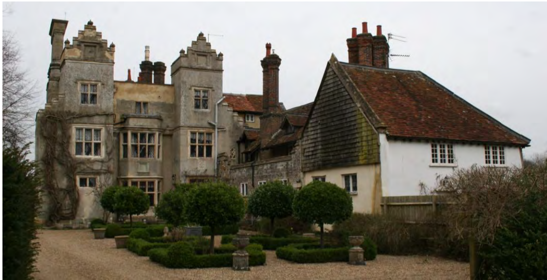
2022. The south elevations.
