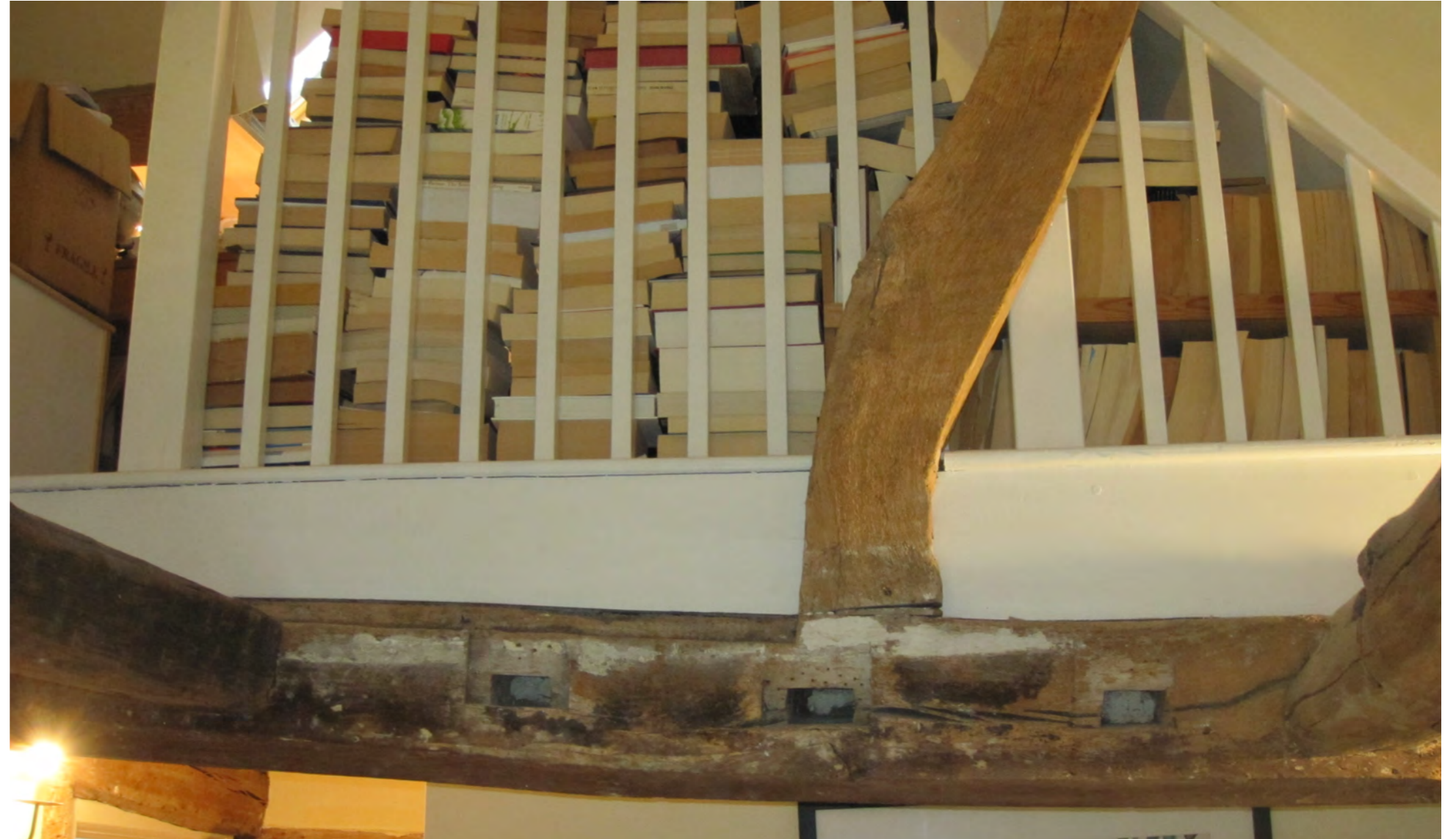
figure 3.1 Mezzanine in master bedroom
