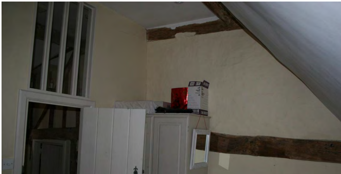
The continuation of the collar and tie-beam seen in Bedroom 1.
