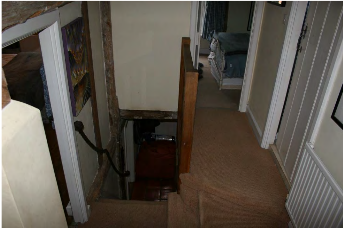
Looking S over the stairwell.
