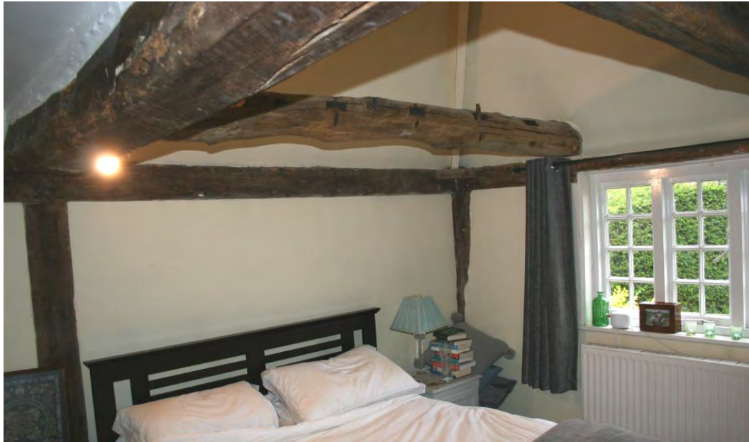
Looking E in Bedroom 2. A fake frame has been affected.
