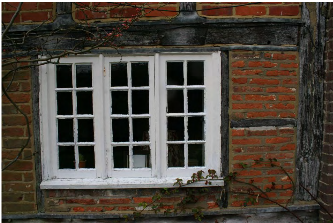
The lower register has thin 'Tudors' as well a larger bricks.
