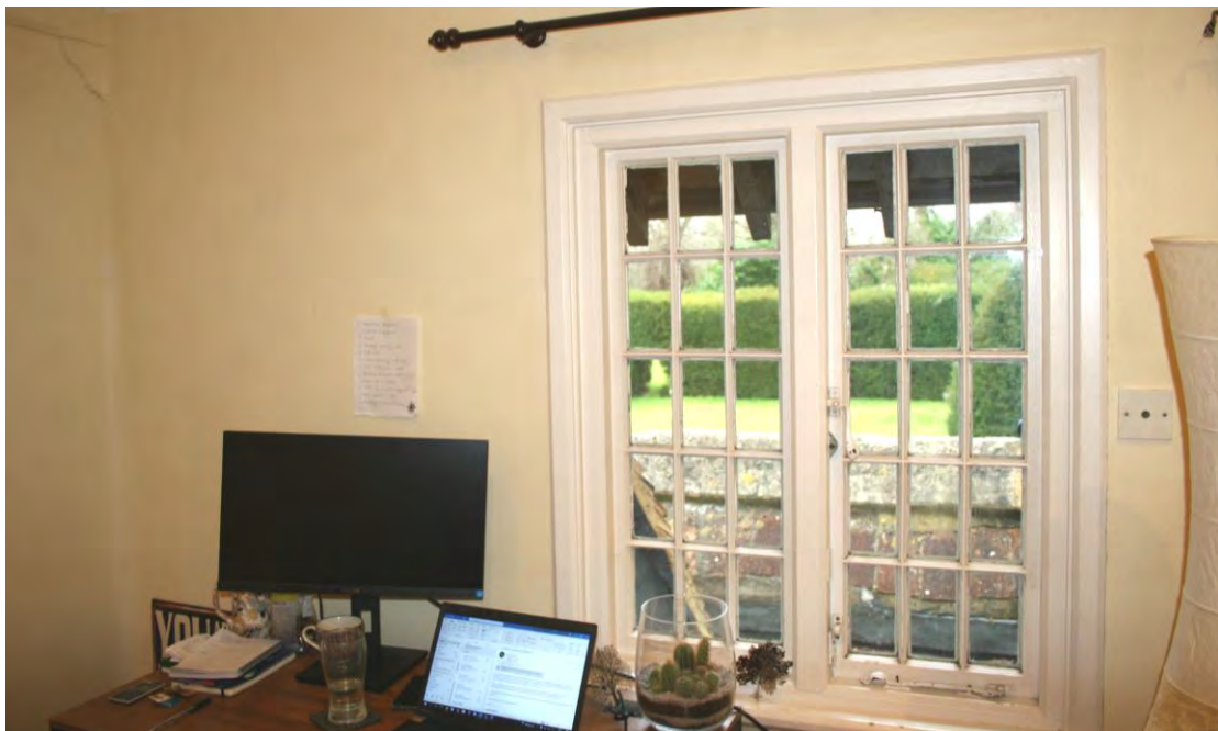
The window in Bedroom 3 allows access to the roof gutter. Looking W.
