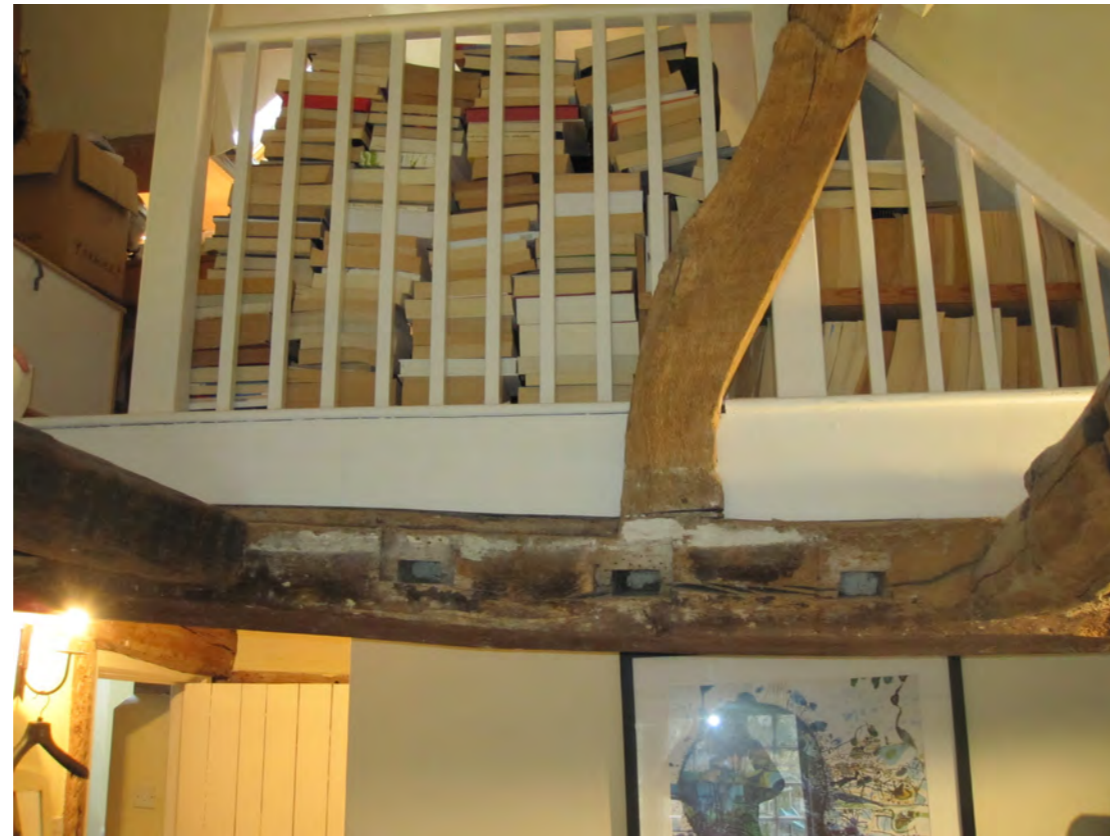
figure 2.4 beams around mezzanine, with plasterboard partition to en-suite below
