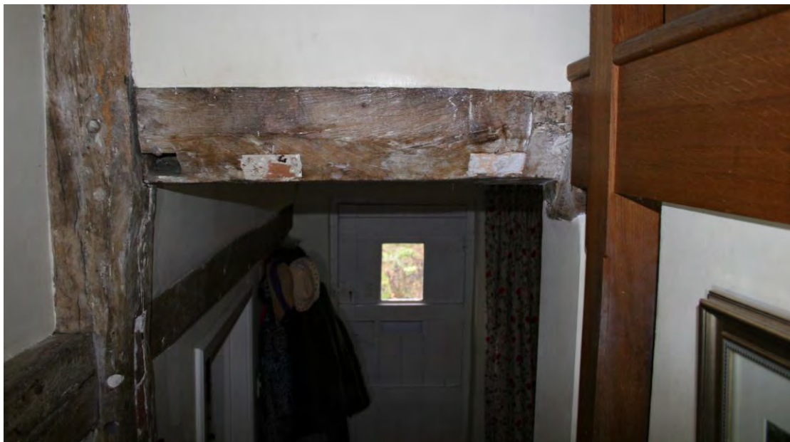
The midrail has been raised to insert the stairs.
