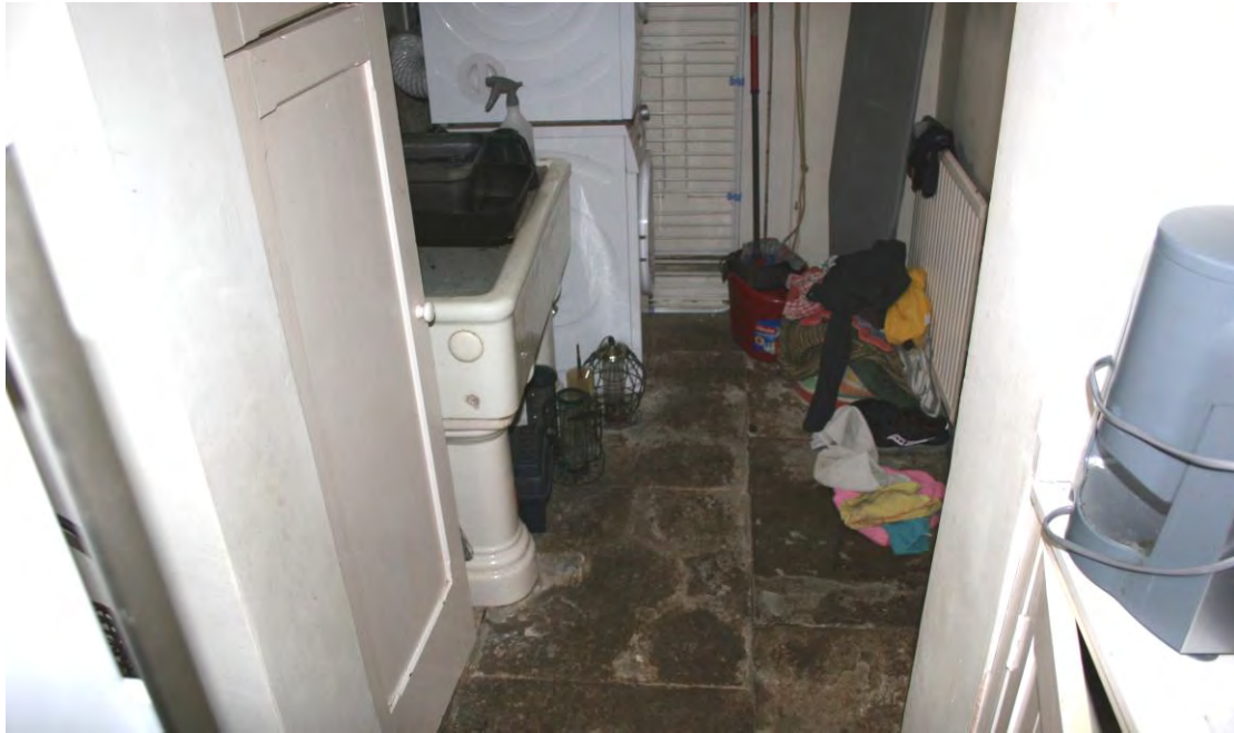
Looking N into the Utility Room.
