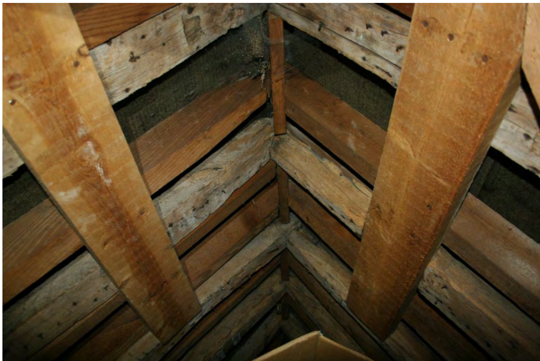
The apex of the cross-wing roof with modern reinforcement. Looking W.
