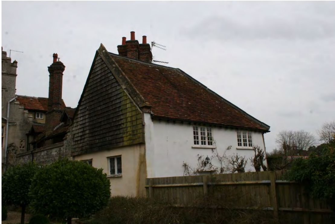
The west and south elevations.
