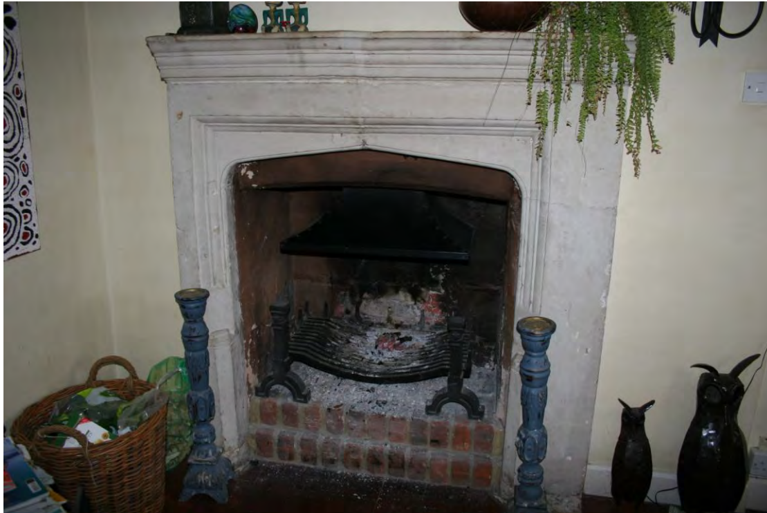
Stone fire surround with cement rendered brick fireback.
