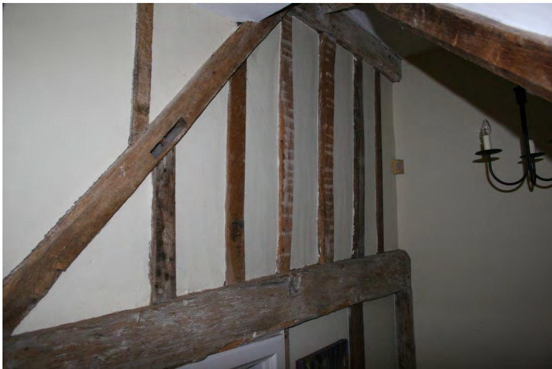
Exposed reused timbers over the stairwell.
