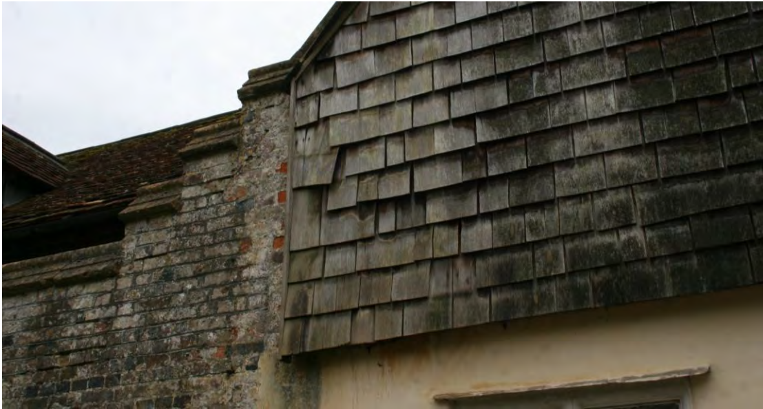
Detail of the shingles.
