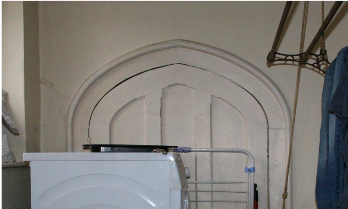
The connecting door to the rest of the Range. Looking N.
