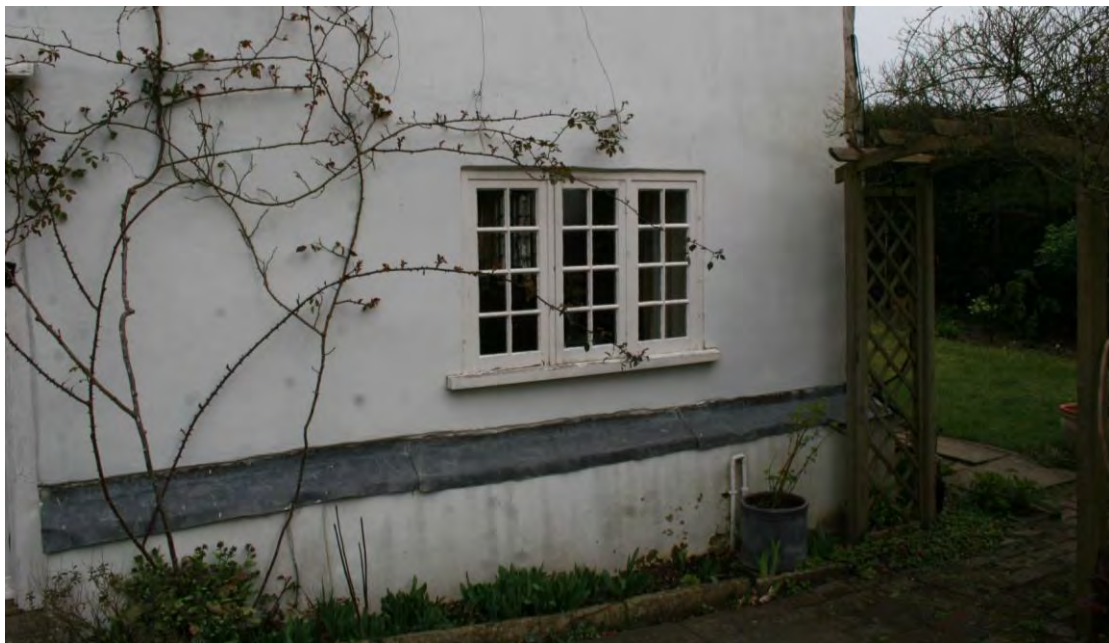
Detail of the inserted window.
