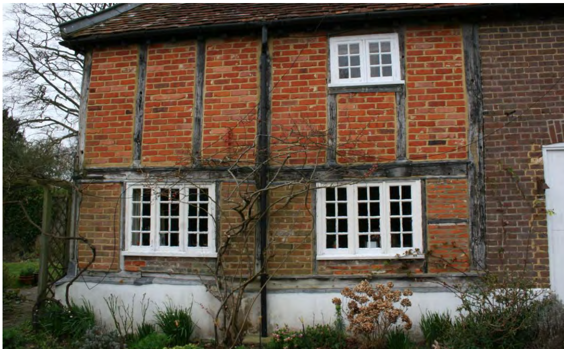
Detail of the LC20th brick panels.
