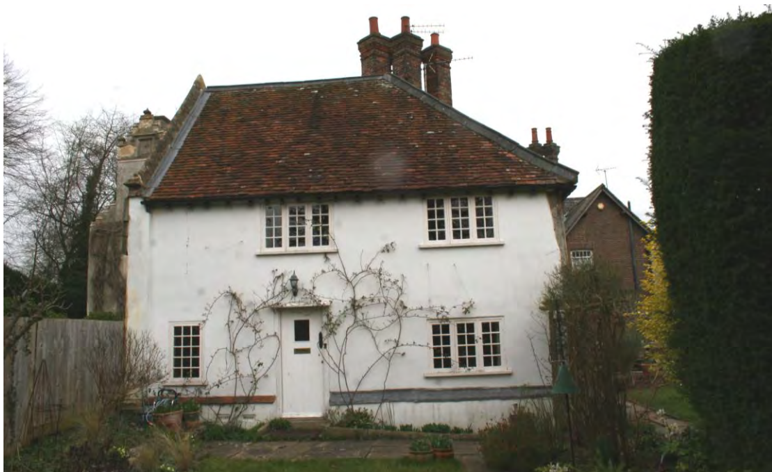
The south elevation of the cross-wing.
