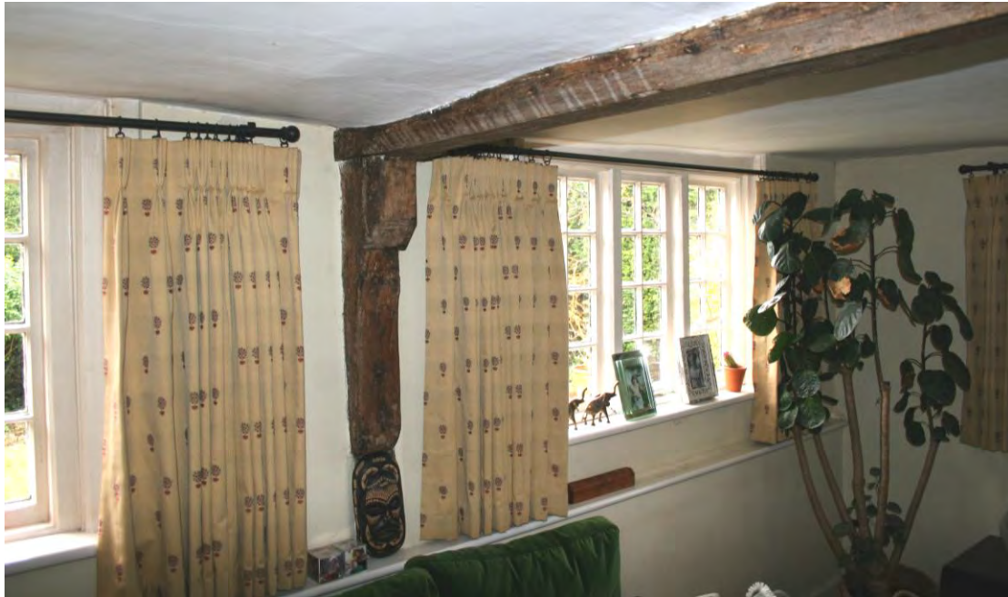
The storey post with applied jowl. Looking SE.
