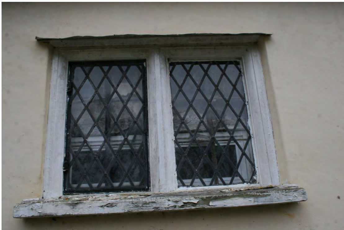
Detail of the southern leaded light window.
