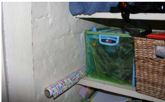
Solid brick wall for the closet.
