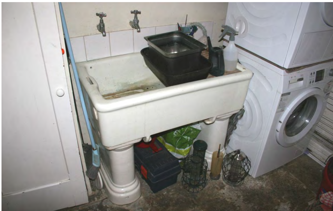
Victorian style butler sink.
