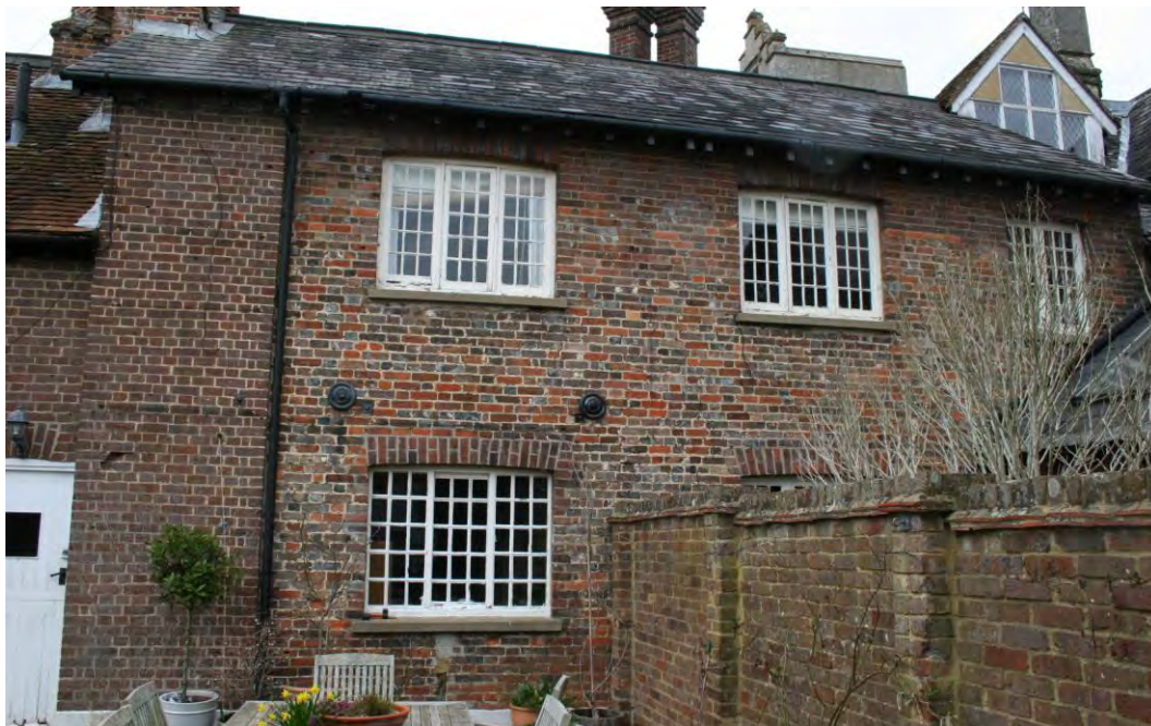
The Range appears to have C18th brickwork with MC19th details.
