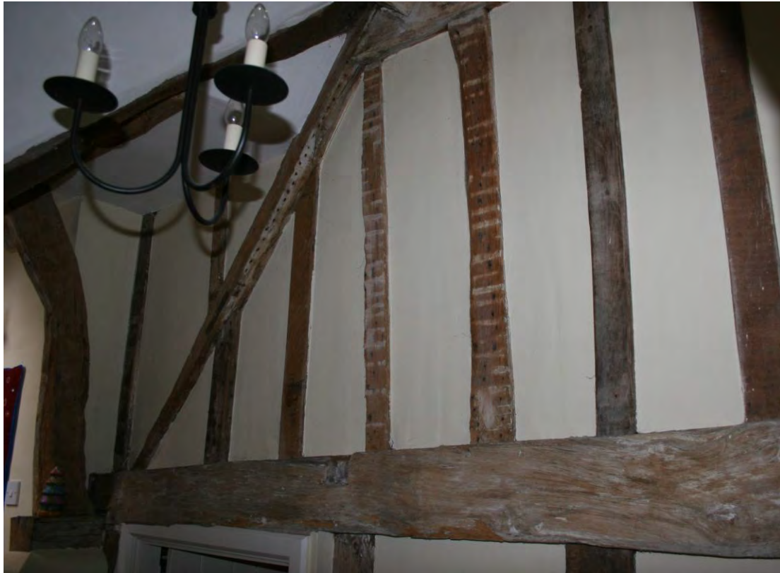
The principal rafter and tie-beam looking NW.
