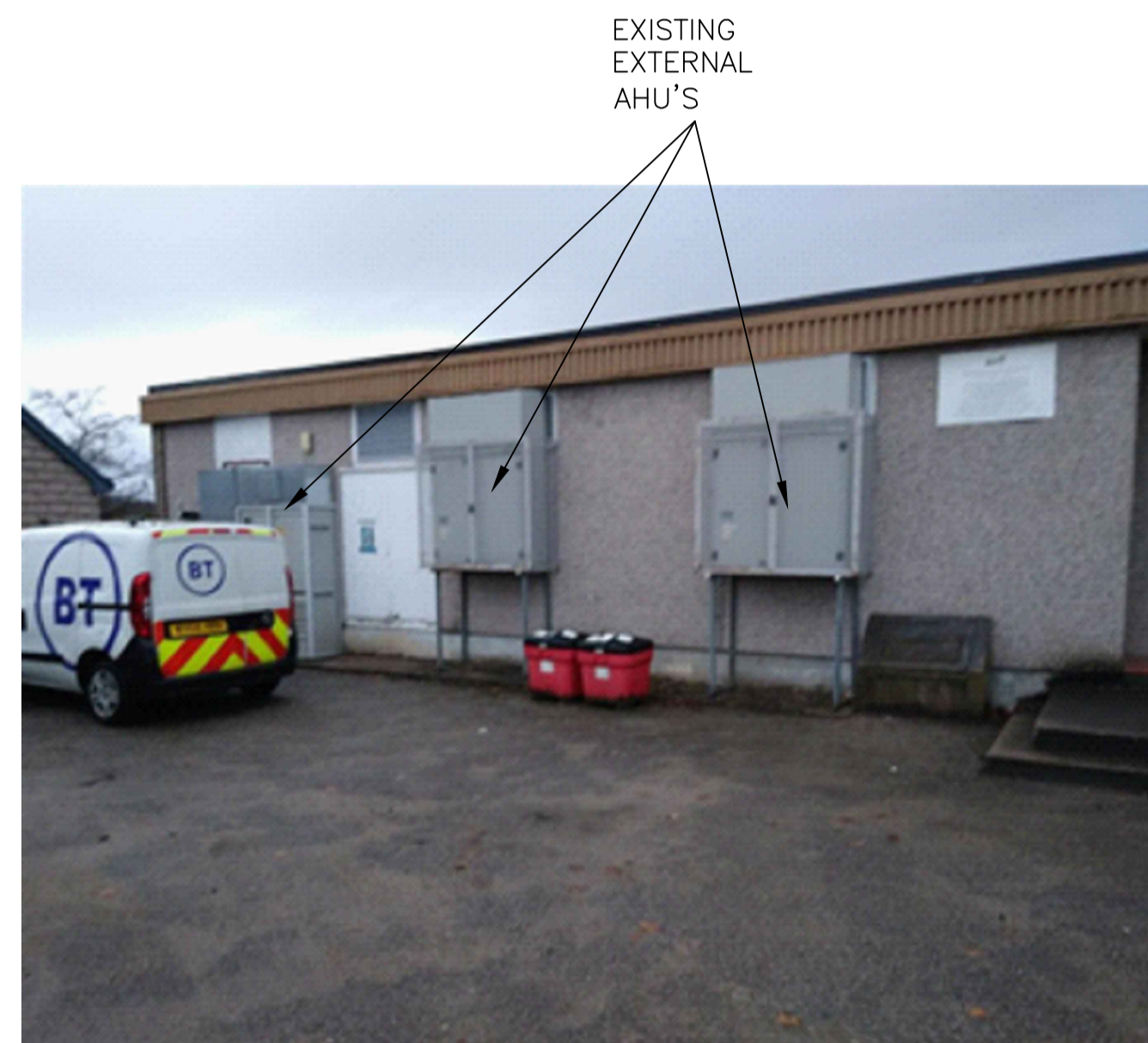
PHOTO OF NORTH ELEVATION
