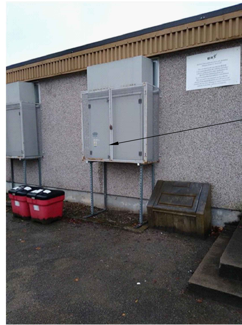
PHOTO OF NORTH ELEVATION
