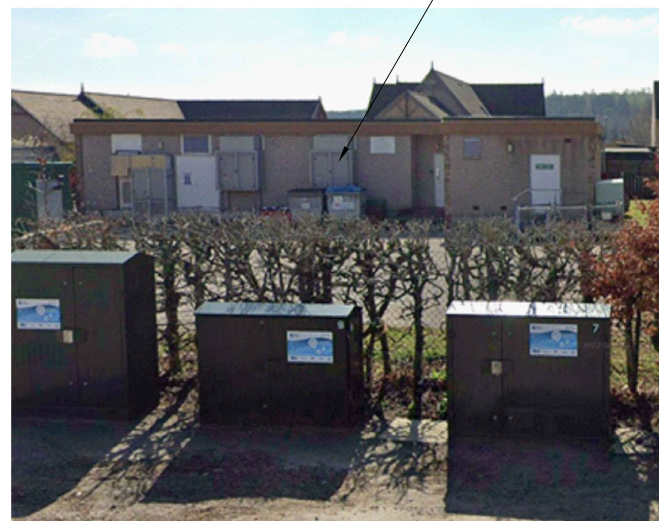
PHOTO OF NORTH ELEVATION
