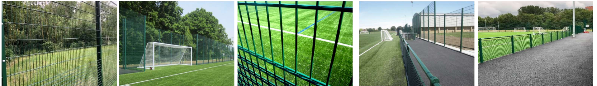
Rigid panel ballstop fencing to perimeter of facility, powder coated dark green to be discrete against a rural backdrop
