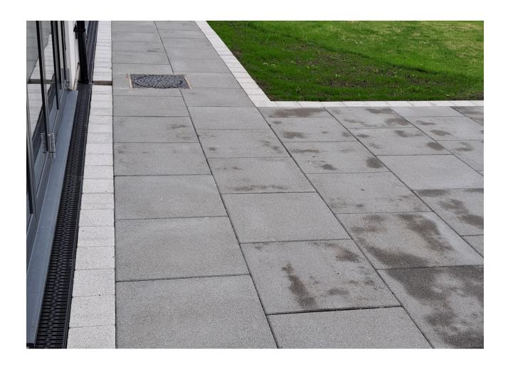
Paving to Main driveway entrance: Tobermore pavers with no mortar joint with white Tobermore pavers with no mortar joint to borders.
