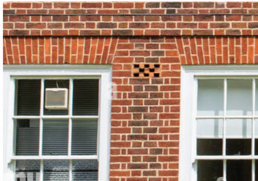
1. Sash window detailing in red brick
