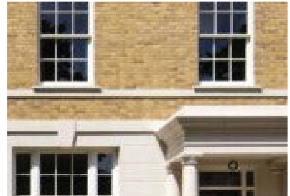
2. Yellow brick with rusticated plinth
