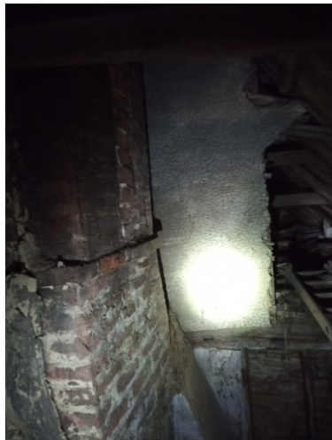
d. Loft space above the secret room.
