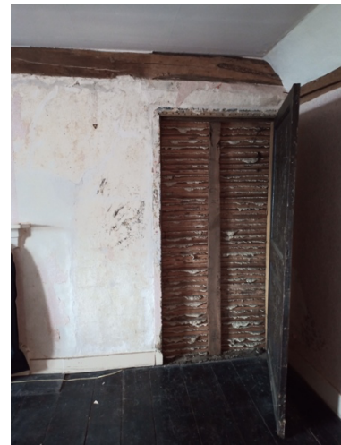
f. Blocked doorway between the secret room and Bedroom 1.
