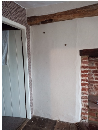
a. Location of the original opening.
