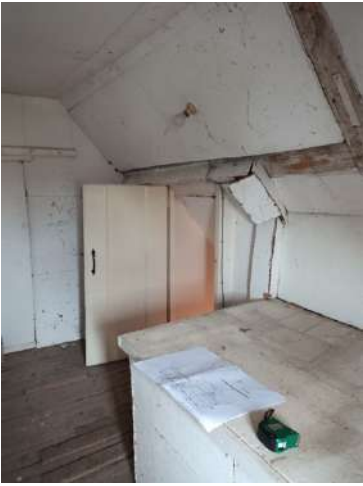
Loft space – East side
