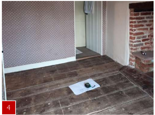
Main house. Bedroom. Well preserved 230mm floorboards
