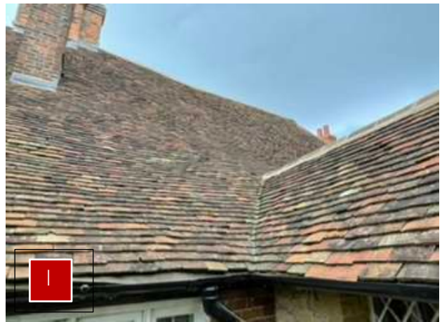
Main house. Historic Roof Junction
