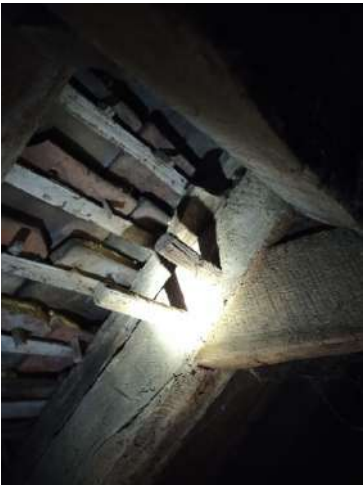
Roof space Left – Kent peg roof tiles – pegs still present Center – Central chimney stack Right – Void due to collapsed joists
