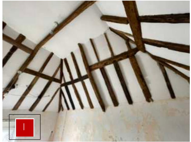
Main house. Original timber frameing with oak purlins and rafters
