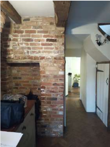
East side entrance area
