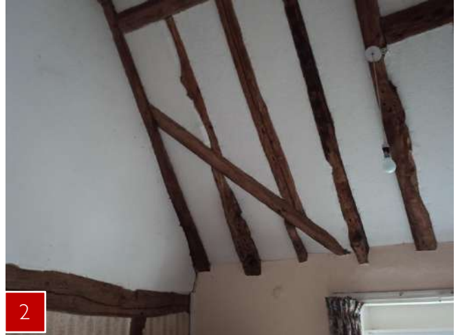
Main house. 18th century extension. Timber from the main house most likely used for the roof structure.
