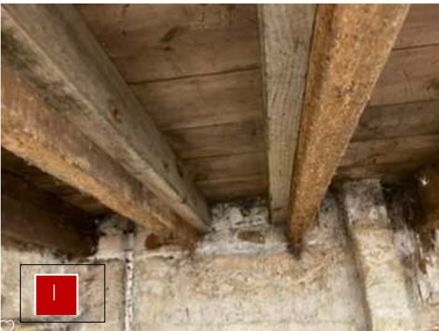
Main house. Basement- Histoirc beams supported by later C20 Timber supports.
