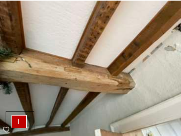
Main house. Original Beam
