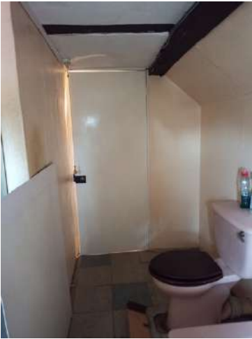
Bathroom/en-suite to Master bedroom facing East
