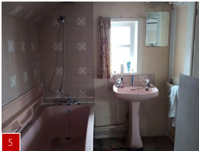
Main house. Bathroom roof includes historic timbers
