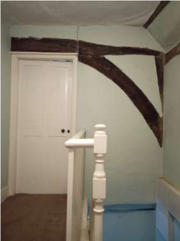
Firstfloor – west side staircase and landing
