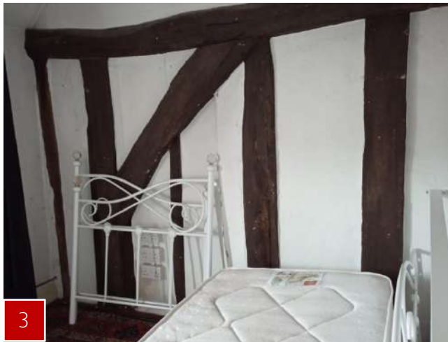
Main house. Bedroom. 17 th century house braces and diagonal
