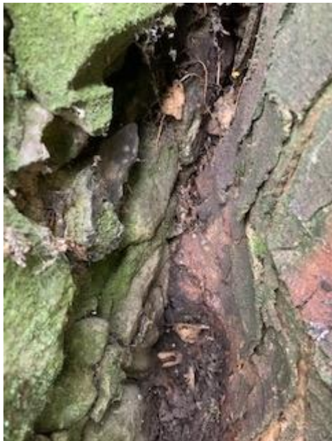
Tree lifting and pushing wall out of line
