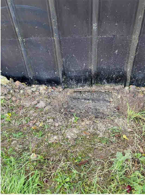
Photograph 16: Trial Hole on Column Foundation, North Elevation.
