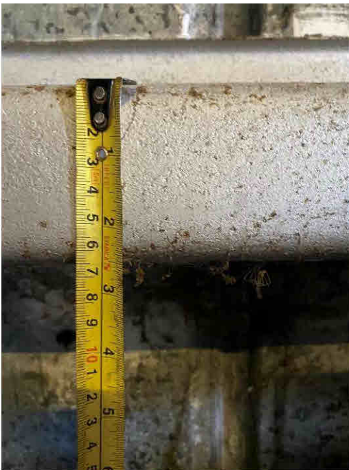
Photograph 15: Cladding Rail Flange Width Measured at Approximately 65mm.
