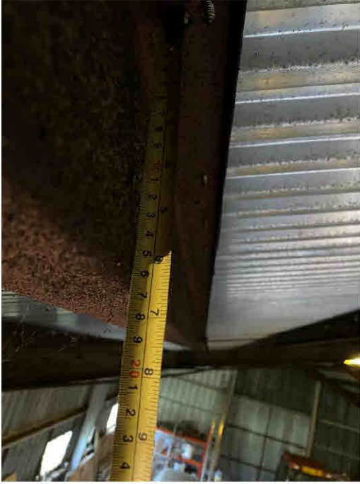
Photograph 8: Purlin Depth Recorded as Approximately 150mm. Note Surface Corrosion to Purlin.
