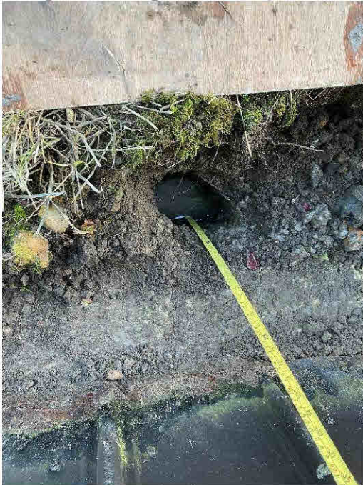
Photograph 18: Pad Foundation Projects Approximately 250mm From Face of Cladding Indicating 900mm Square Pad.
