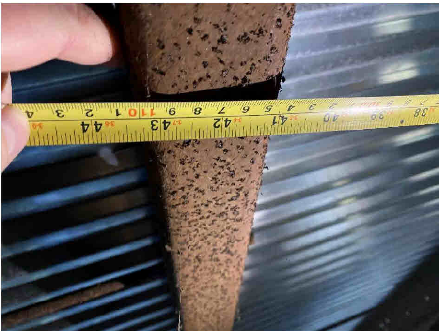
Photograph 13: Purlins Generally at 1050mm Centres.
