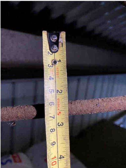
Photograph 11: Crossed Steel Rod Bracing Approximately 10mm Diameter.
