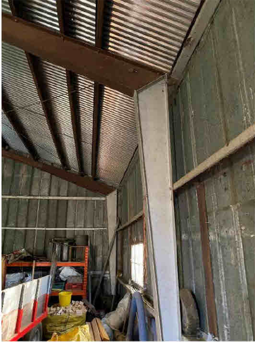
Photograph 4: Typical Portal Frame Column, Note Tapering Profile.
