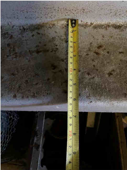
Photograph 14: Cladding Rail Depth Measured as Approximately 150mm.
