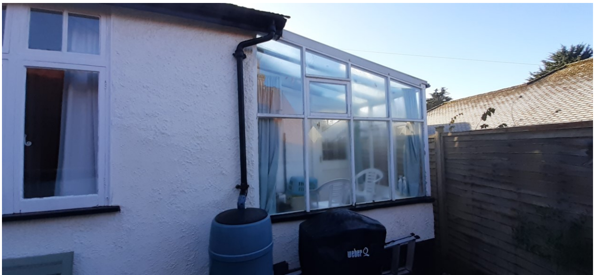
Side / north elevation showing existing rear sun room / conservatory
