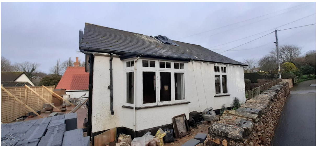
Side / south elevation showing car port and rear lean-to demolished.
