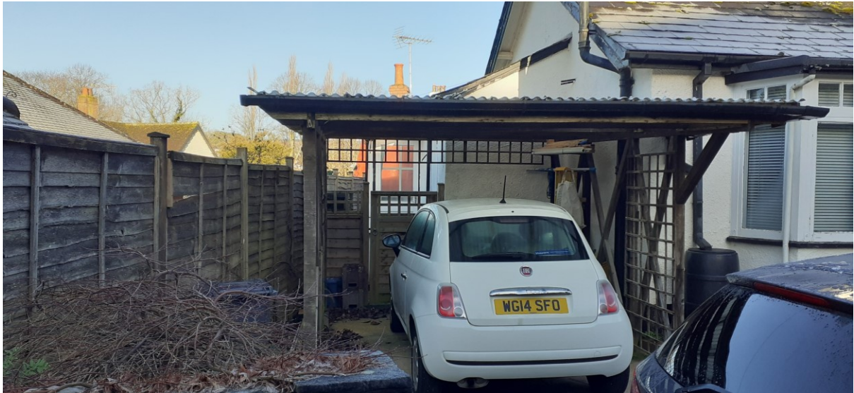
Side / rear elevation showing existing car port and rear lean-to.
