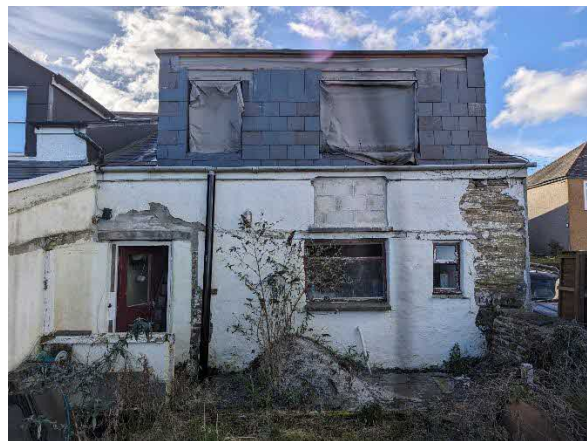
Photo 2. Showing the rear of the house and new dormer from the east
