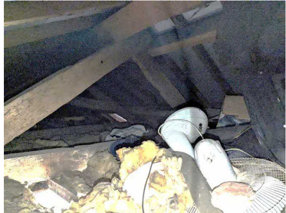
Photo 4. Showing the roof void
