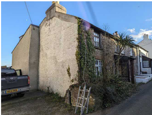
Photo 1. Showing the front and northern gable end of the house
