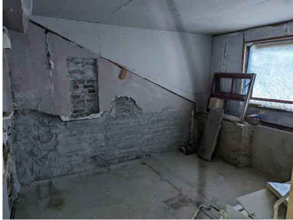
Photo 3. Showing the interior of the new rear dormer
