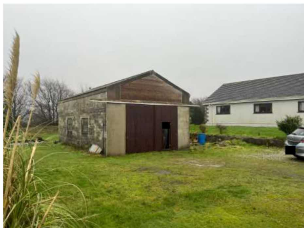
Photograph 1. North and west elevations.
