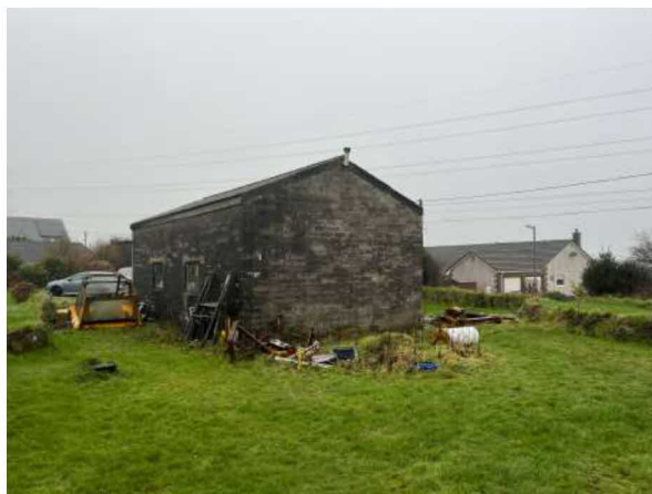
Photograph 2. East and south elevations.
