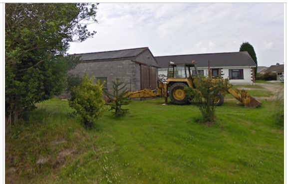
P.2 Existing Garage
