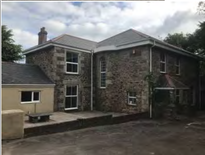
Plate 6: A view looking northeast at the main part of the dwelling/building.
