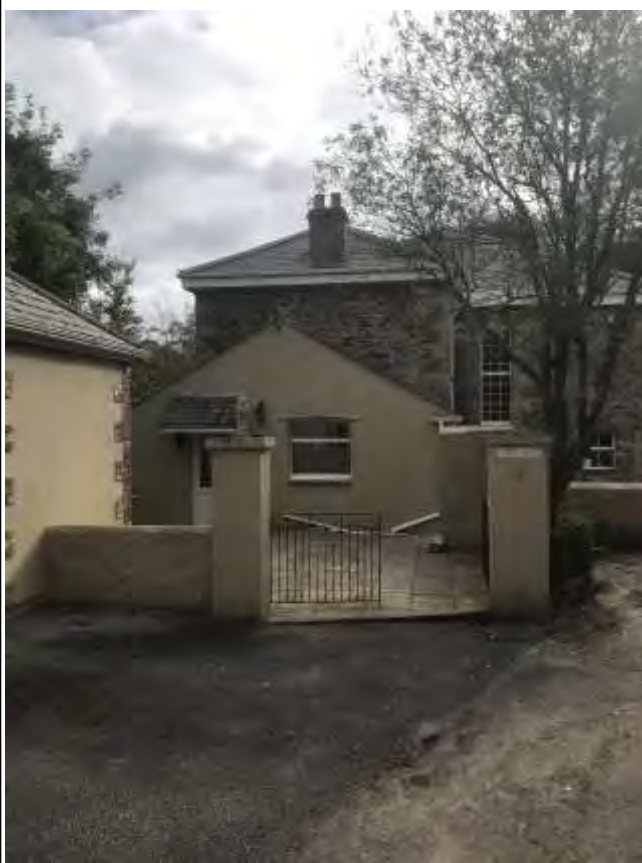
Plate 5: A view looking towards the east. The original stone built part of the building is in the background and in the foreground is the modern single storey extension.
