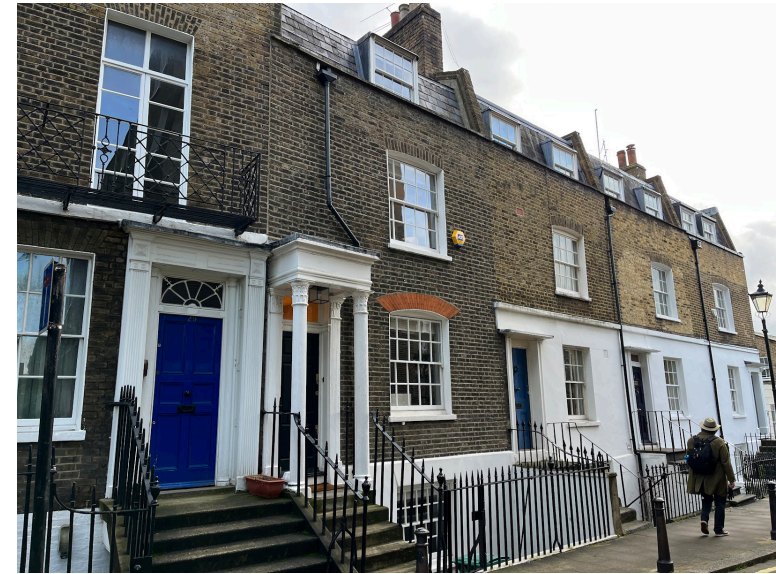
Plate 1 View of the site's principal and flank facade in the context of its wider listed terrace.
