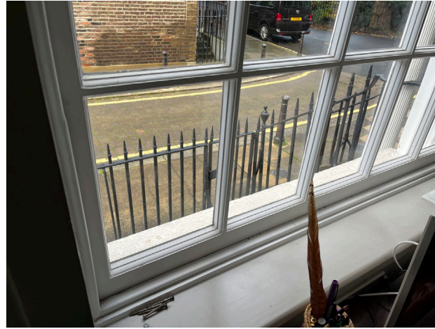
Plate 4 Modern glazing to front facade.
