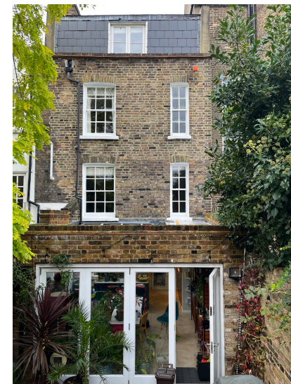
Plate 2 View of site's modern rear full height extension and boundary wall.
