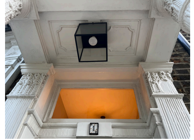
Plate 5 Historic fluted pilasters and mouldings to soffit to entrance porch.
