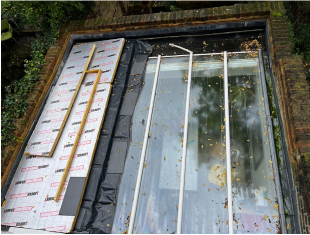
Plate 3 View of modern glazed roof to 2010 extension.
