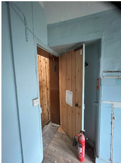
Door to existing side stairs to retail shop below. Opening to be blocked up, stairs removed.
