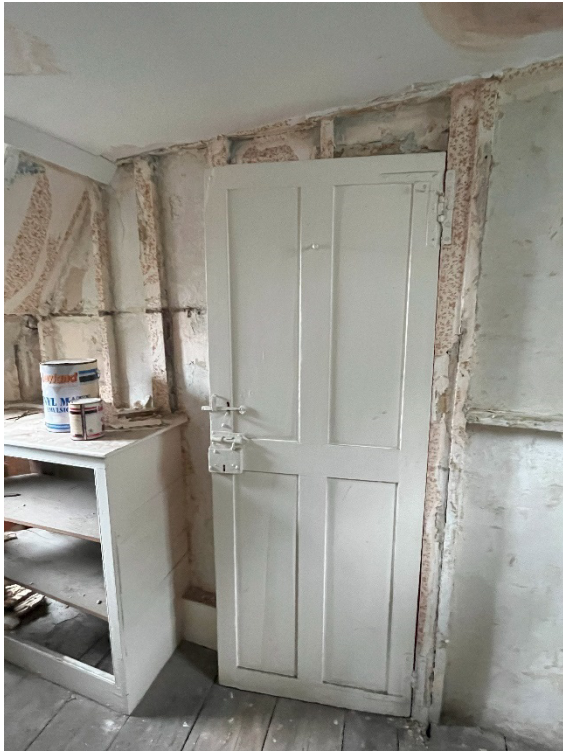
Door to bathroom area from Hall and stairs.
