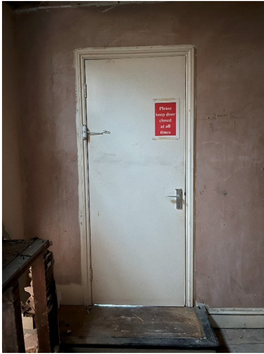
Door from kitchen area to rear bedroom. To be replaced with panelled door.
